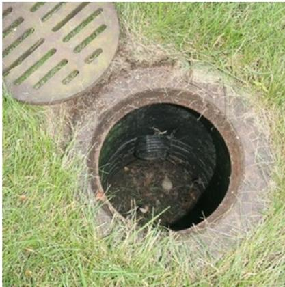
Dry well use is applicable only where their subgrade soils have the required permeability rates. Like other BMPs that rely on infiltration, dry wells are not appropriate for areas where high pollutant or sediment loading is anticipated due to the potential for groundwater contamination. Specifically, dry wells must not be used in the following locations:
