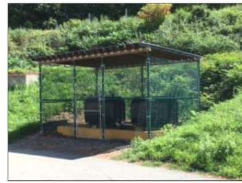
Used Oil Storage Containment Area
