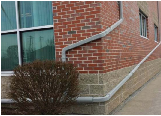
Photo: Downspouts at NBC's Corporate Office Building
