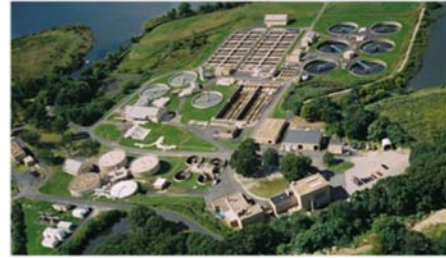
Photo: Bucklin Point Wastewater Treatment Facility
