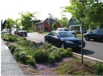
Photo: Example of Green Stormwater Infrastructure
