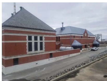
FPWWTF Ernest Street Pump Station
