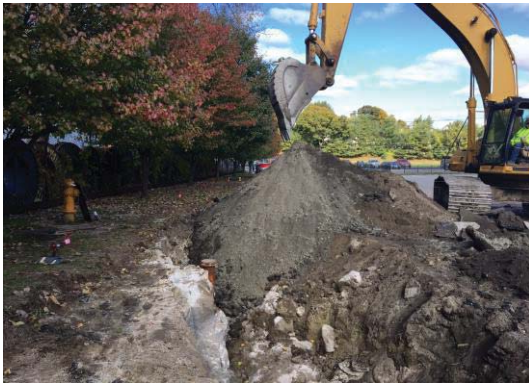
Photo: Construction on the Moshassuck Valley Interceptor
