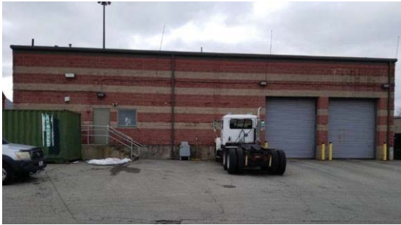
Photo: Sludge Dewatering & Handling Facility
