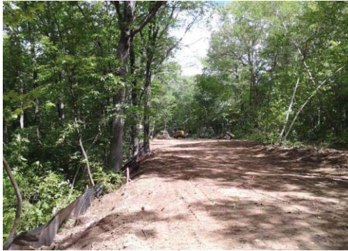
Photo: Easement clearing
