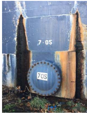
Photo: Secondary Digester
