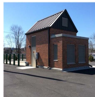
Photo: WCS01 Gate & Screening Structure
