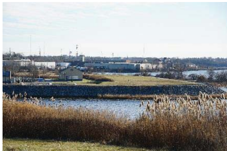
Photo: Bucklin Point WWTF
