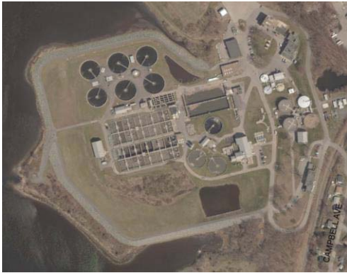
Photo: Existing Clarifiers at Bucklin Point
