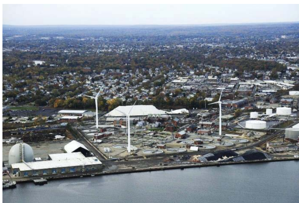
Photo: Field's Point Wastewater Treatment Facility
