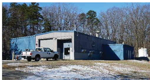
Lincoln Septage Station
