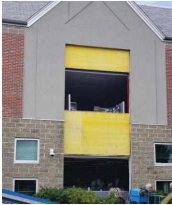
Photo: Window Replacement at COB
