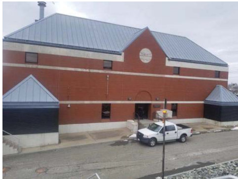
Photo: Ernest Street Pump Station
