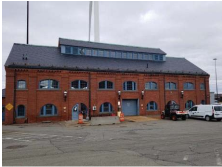
Photo: Existing FPWWTF Maintenance Building
