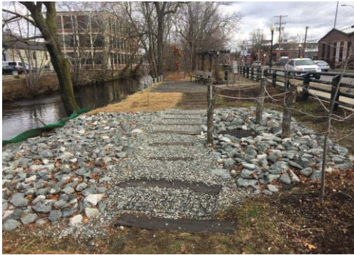
Photo: Surcharge area at Kinsley Ave, Providence
