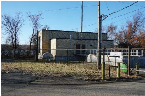
Photo: Omega Pump Station
