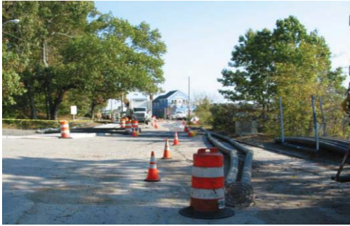
Photo: Rehabilitation of Interceptors
