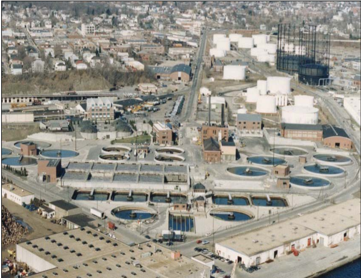
Aerial View - Field's Point Wastewater Treatment Facility
