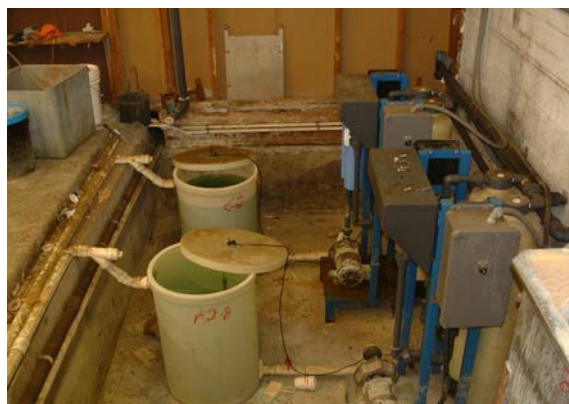
Facility Shutdown Inspection of an electroplating facility that is no longer in operation.
