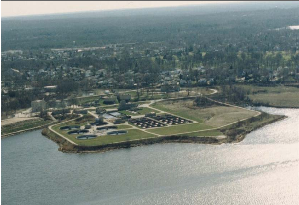
Aerial View - Bucklin Point Wastewater Treatment Facility
