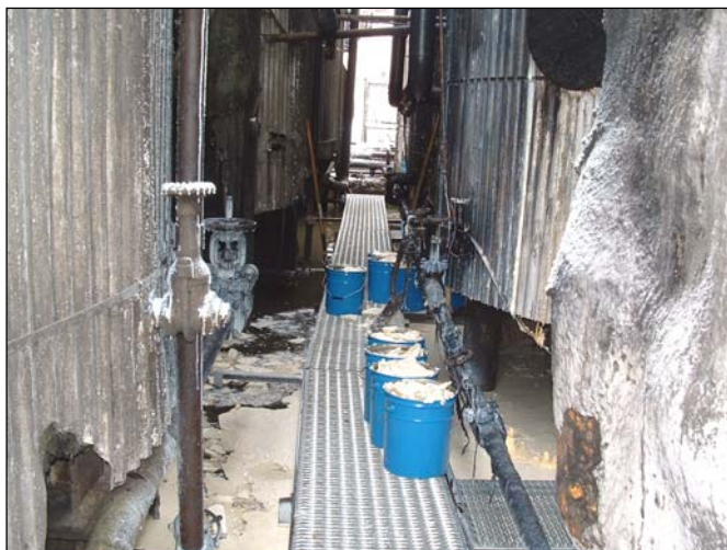
Cleanup underway following a grease spill inside a tank farm at Bunge North America (East)
