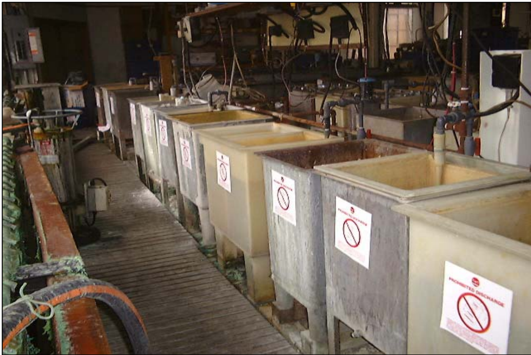
Tanks at a shutdown plating shop are stickered "PROHIBITED DISCHARGE"
