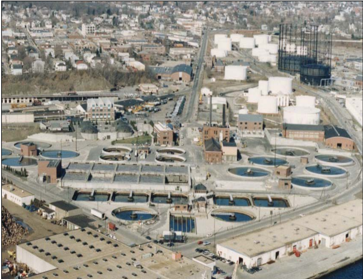
Aerial View - Field's Point Wastewater Treatment Facility
