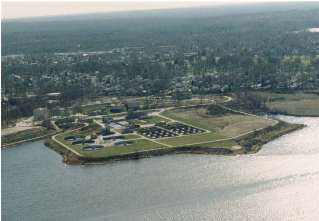
Aerial View - Bucklin Point Wastewater Treatment Facility
