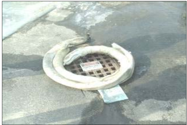
Storm drain at Crystal Thermoplastic protected by absorbent materials
