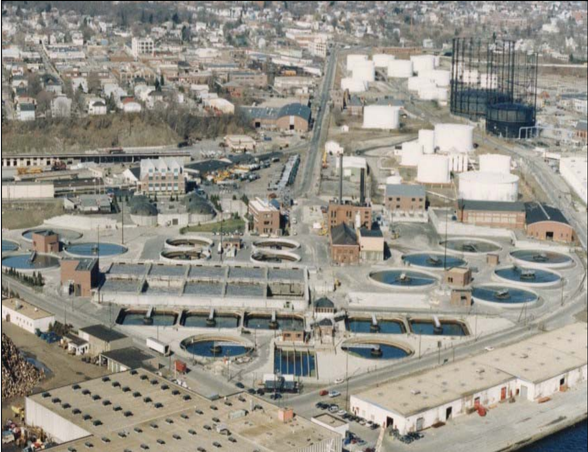
Aerial View - Field's Point Wastewater Treatment Facility
