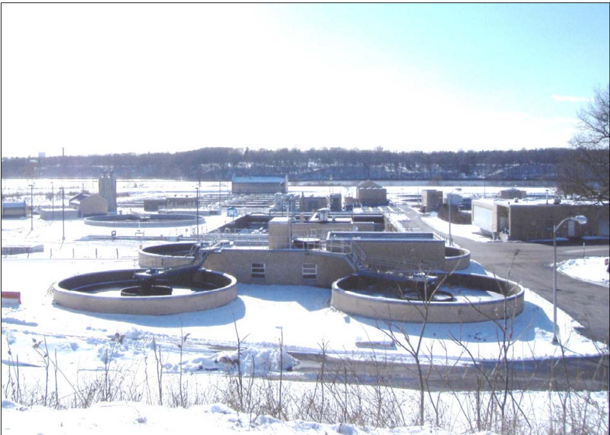
Bucklin Point Wastewater Treatment Facility
