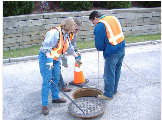
Pretreatment staff investigate an illegal discharge
