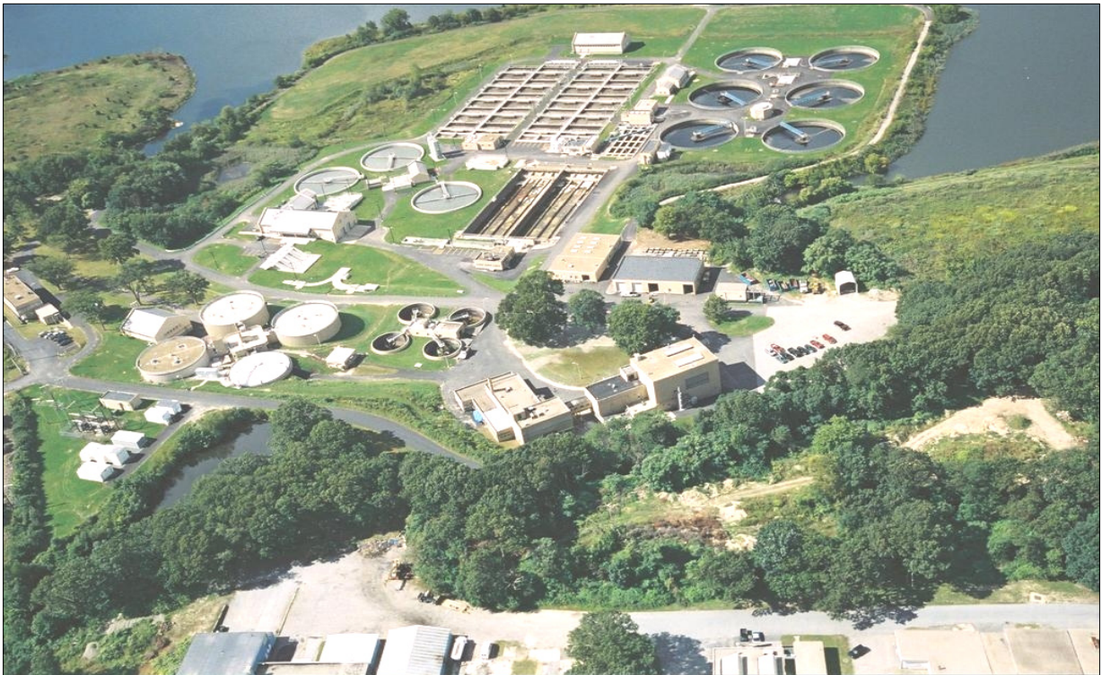
Bucklin Point Wastewater Treatment Facility
