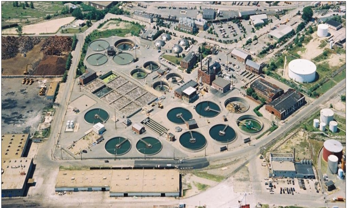
Aerial View - Field's Point Wastewater Treatment Facility
