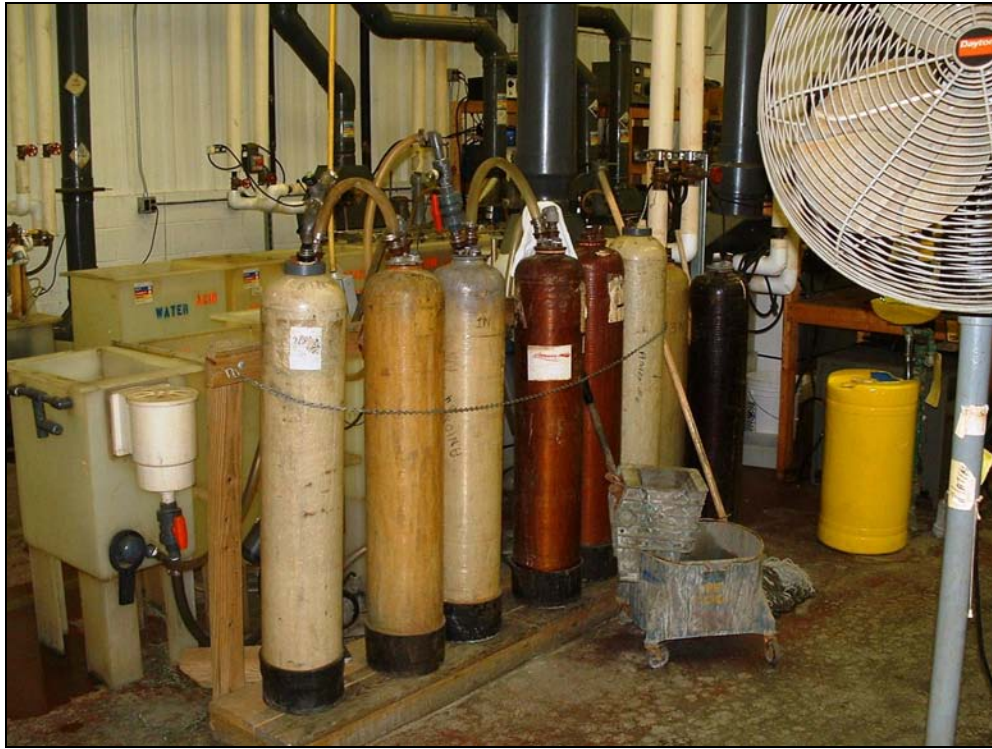
Part of an Ion Exchange System at a Permitted Zero Discharge Facility
