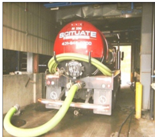
Septage truck discharging at the Lincoln Septage Station
