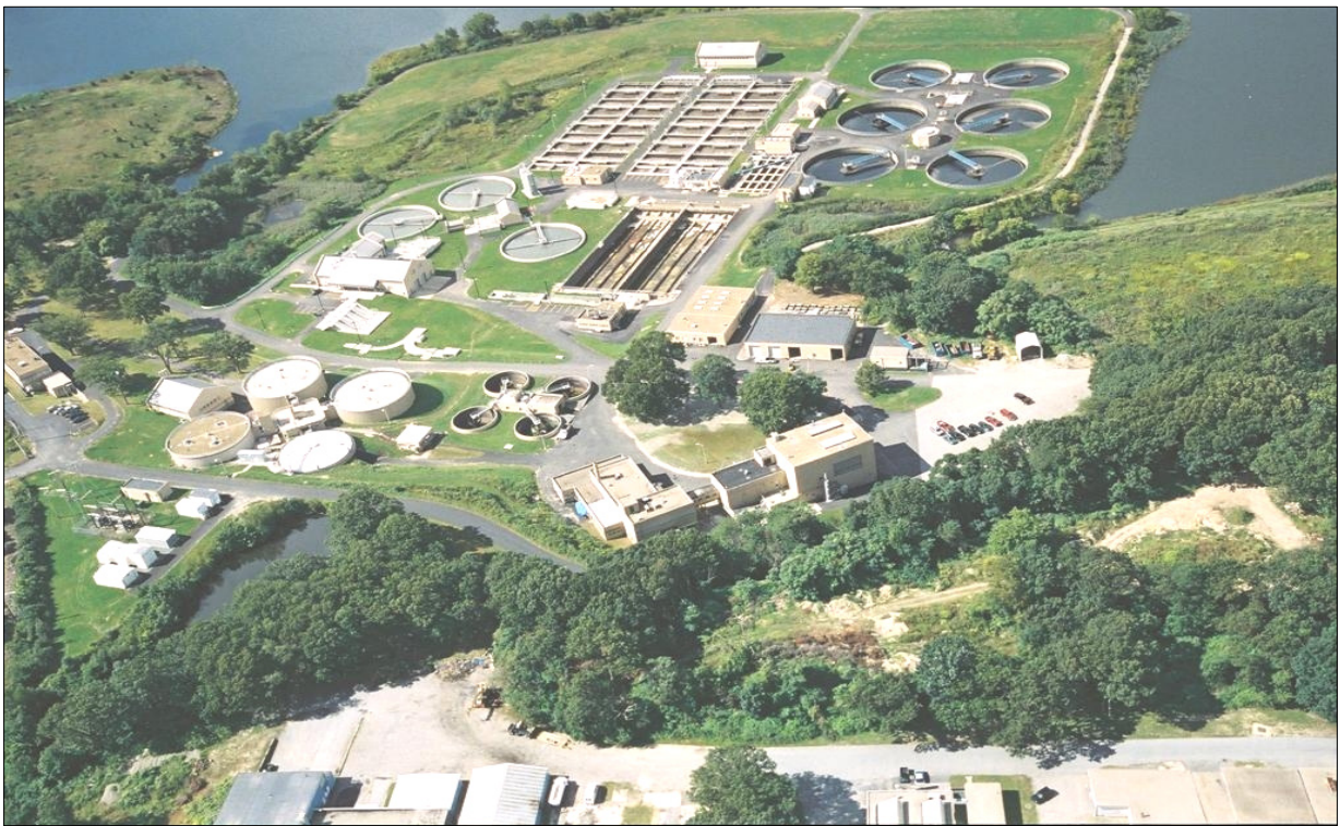
Bucklin Point Wastewater Treatment Facility
