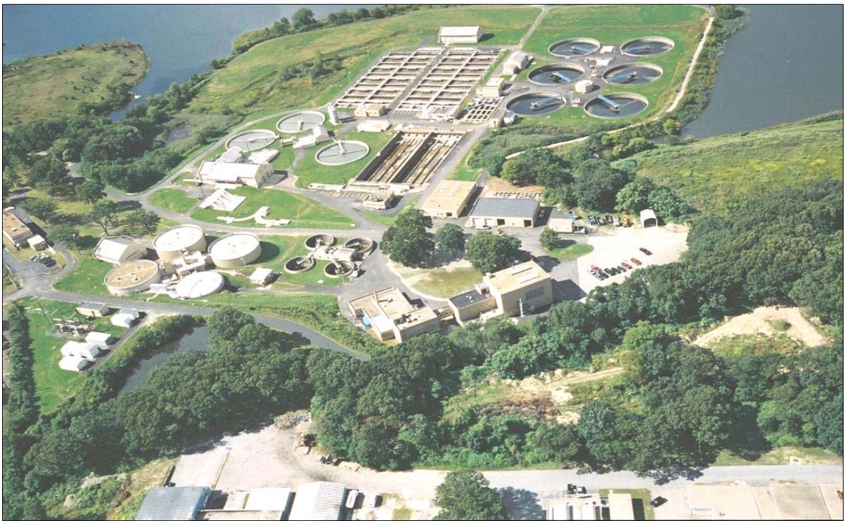
Bucklin Point Wastewater Treatment Facility
