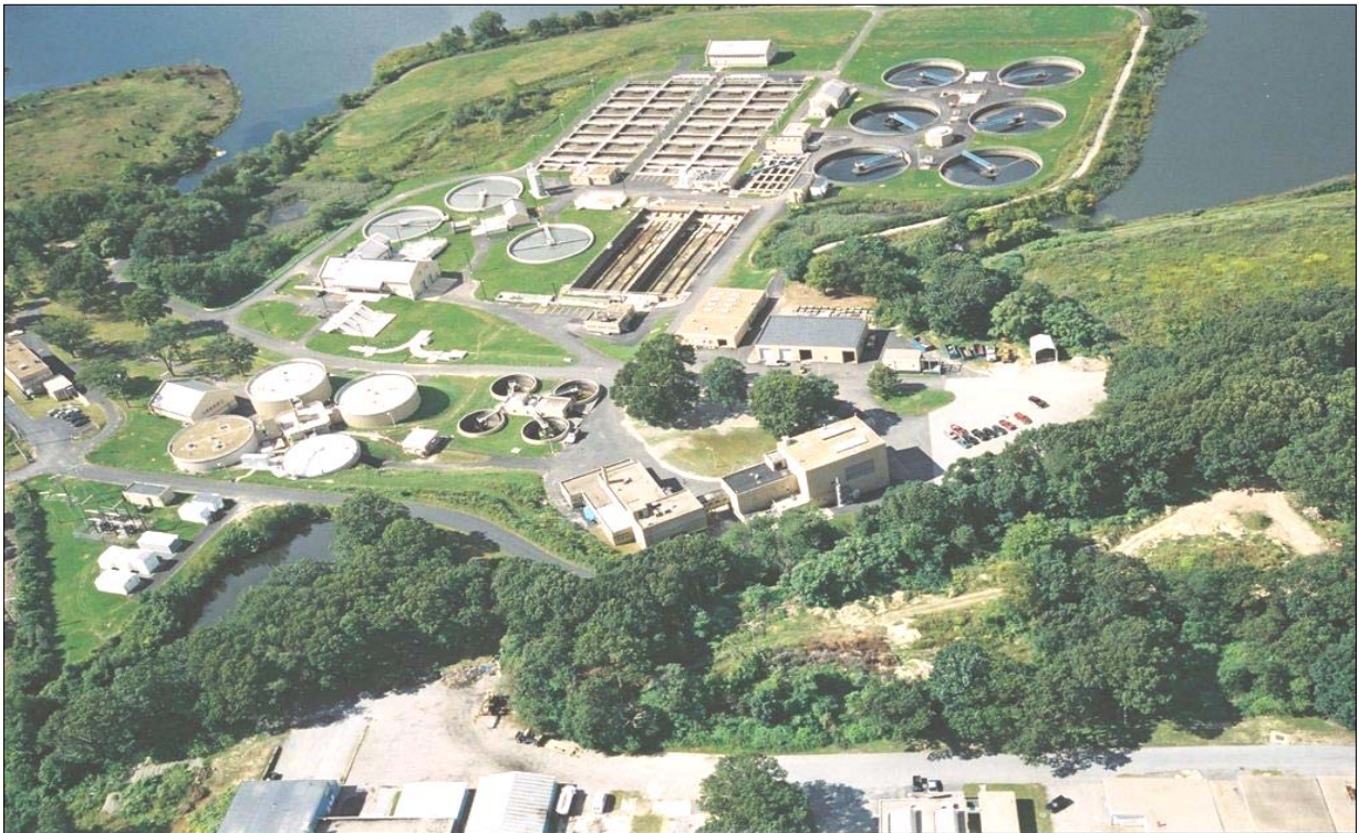
Bucklin Point Wastewater Treatment Facility
