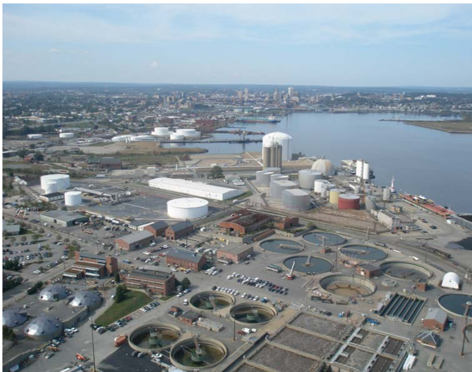
The Narragansett Bay Commission Fields Point Wastewater Treatment Facility. Photo: NBJ.
