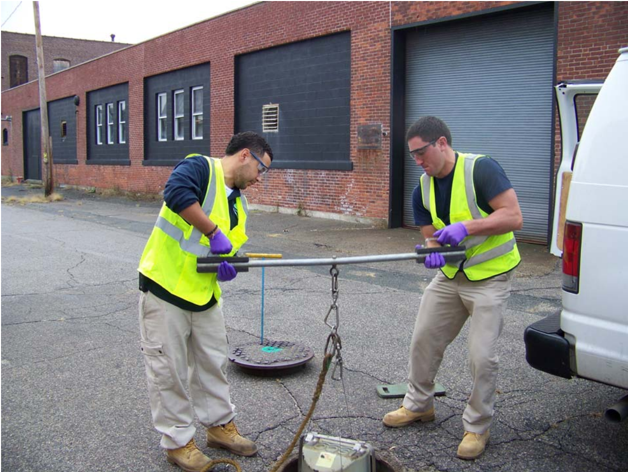
NBC EMDA staff Installing an Industrial Manhole Sampler
