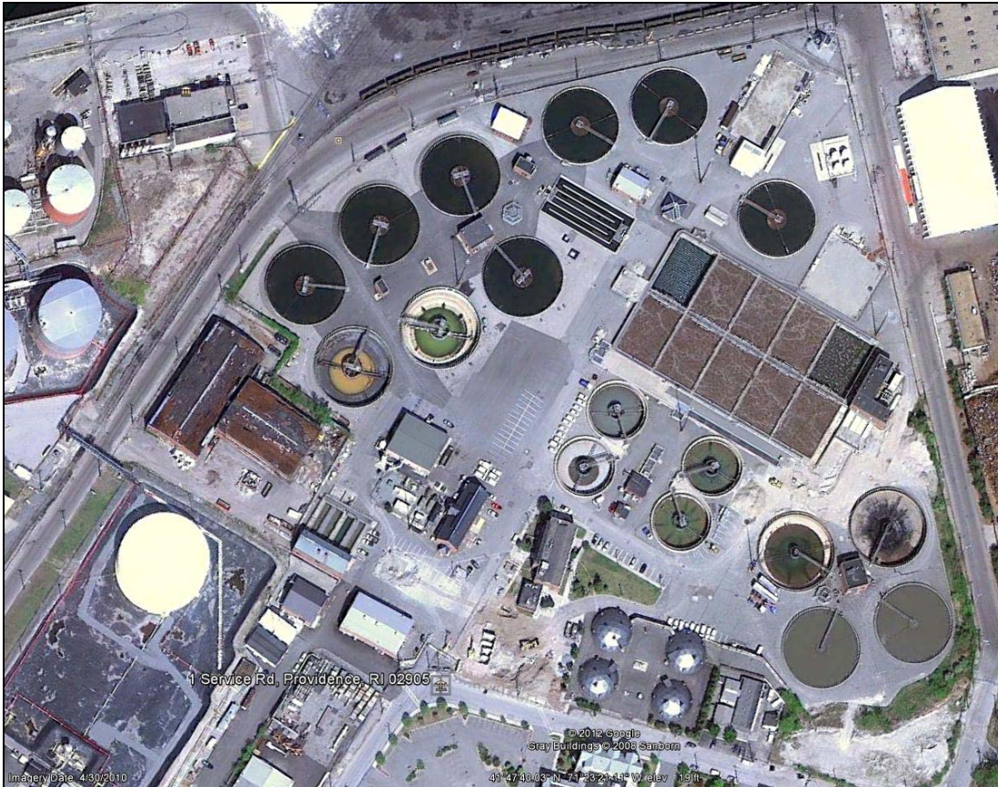
Aerial View - Field's Point Wastewater Treatment Facility
