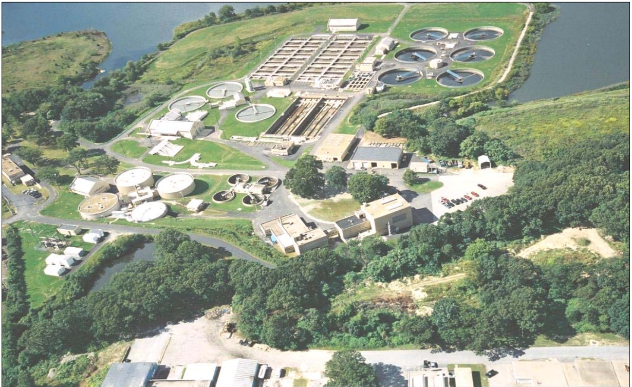
Bucklin Point Wastewater Treatment Facility
