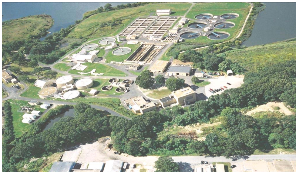
Bucklin Point Wastewater Treatment
