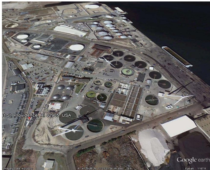
Field's Point Wastewater Treatment Facility
