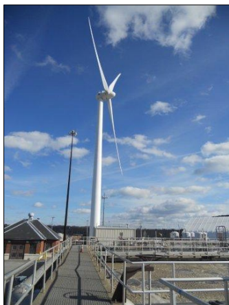
Field's Point Wind Turbine and IFAS Tank
