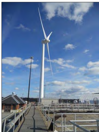
Field's Point Wind Turbine and IFAS Tank
