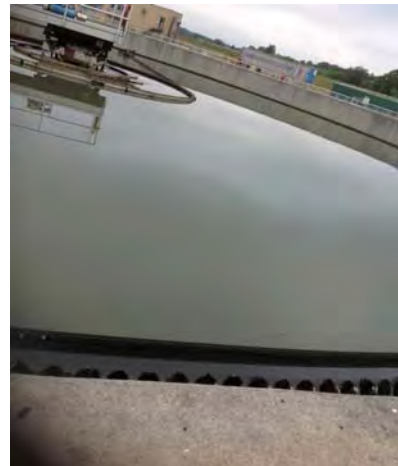
Green Influent at Bucklin Point
