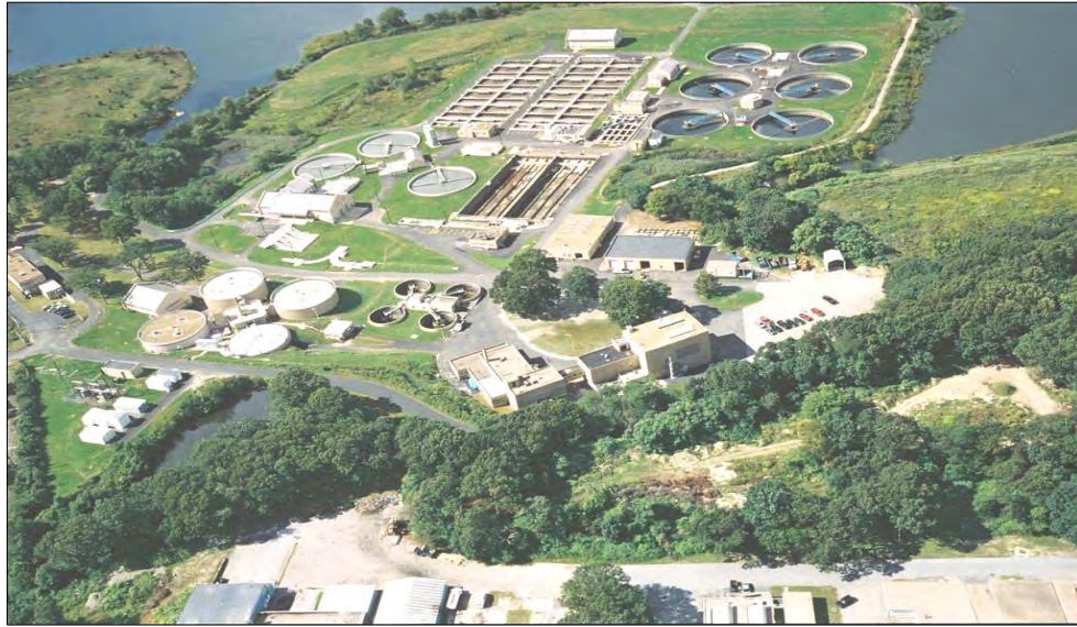
Bucklin Point Wastewater Treatment
