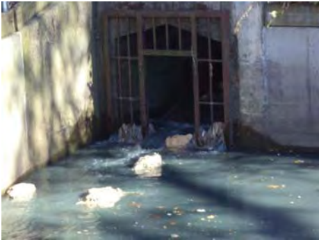
Bucklin Brook Outfall
