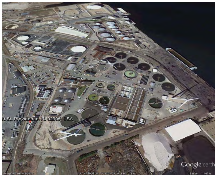
Field's Point Wastewater Treatment Facility
