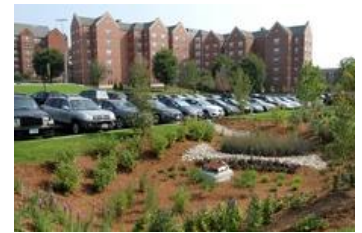
A landscaping feature called a bioswale, tucked next to a new parking lot at Providence College, helps filter out silt and contaminants from stormwater runoff, and also helps educate students about pollution control. The Providence Journal/Steve Szydlowski
