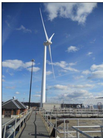
Field's Point Wind Turbine and IFAS Tank
