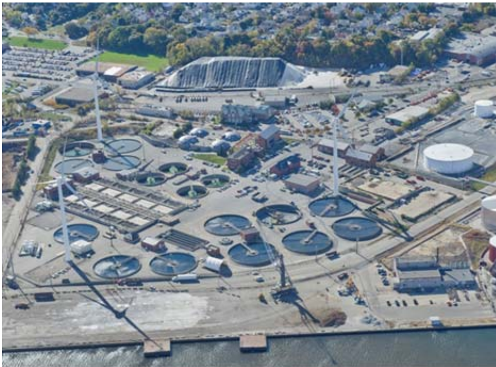
Field's Point Wastewater Treatment Facility
