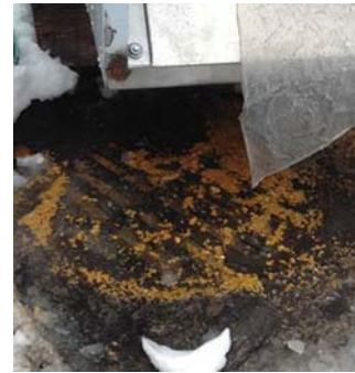
Grease in a Yard Drain
