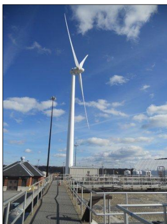
Field's Point Wind Turbine and IFAS Tank
