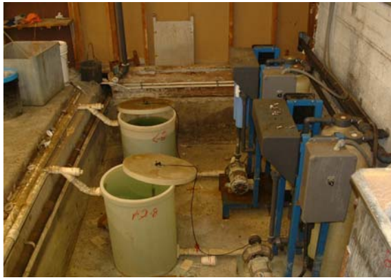
Facility Shutdown Inspection of an electroplating facility that is no longer in operation.
