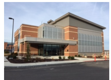
Water Quality Science Building
