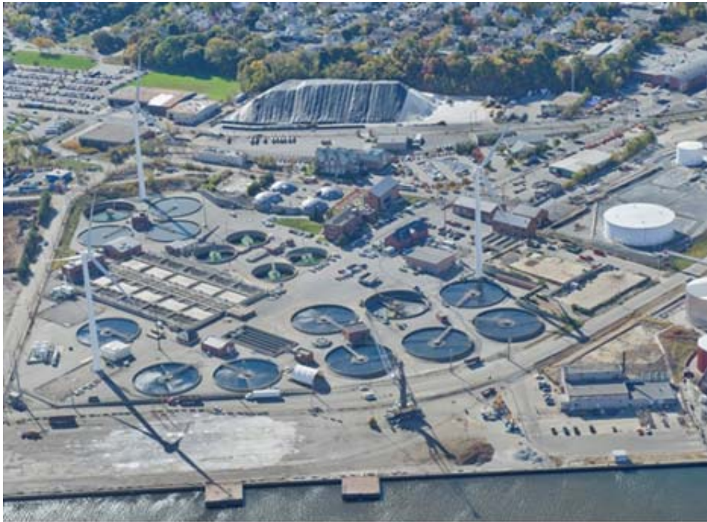
Field's Point Wastewater Treatment Facility
