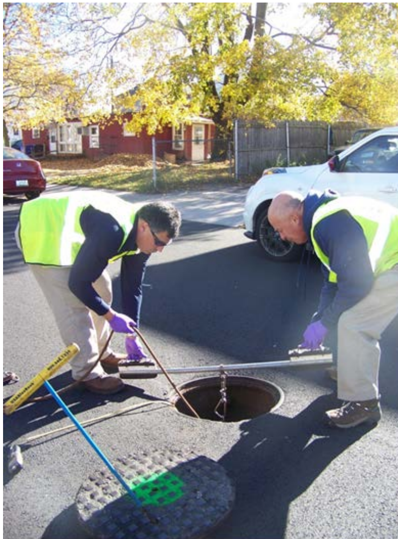
Sanitary manhole sample collection
