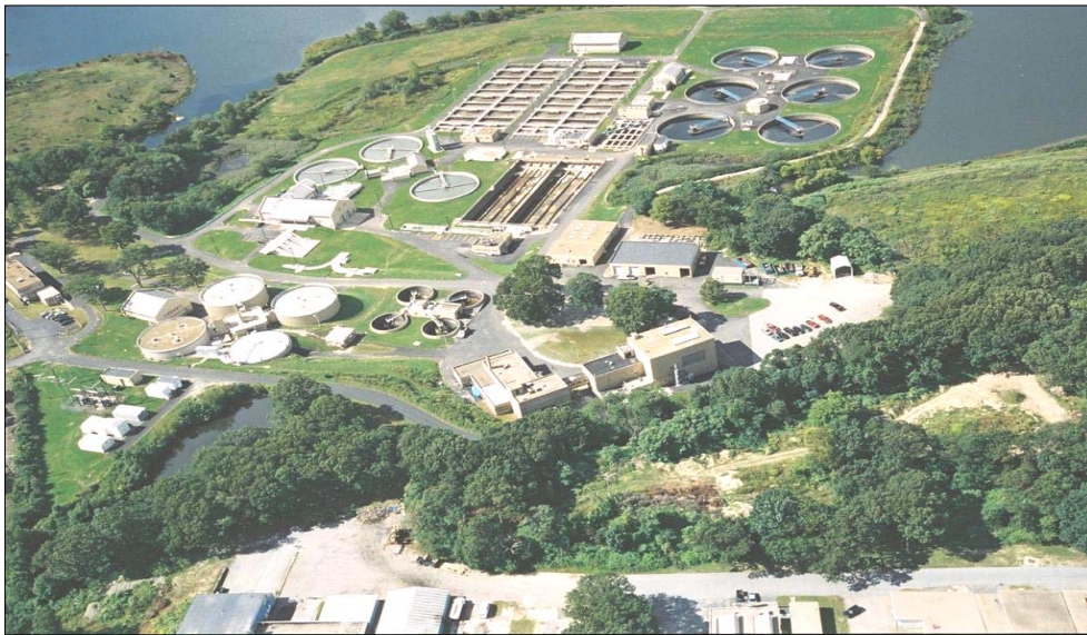
Bucklin Point Wastewater Treatment
