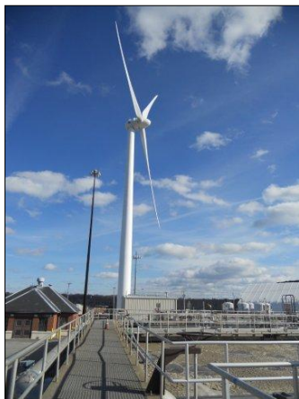
Field's Point Wind Turbine and IFAS Tank
