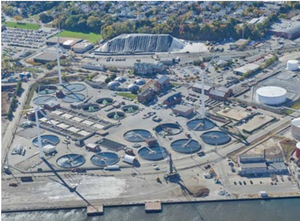
Field's Point Wastewater Treatment Facility
