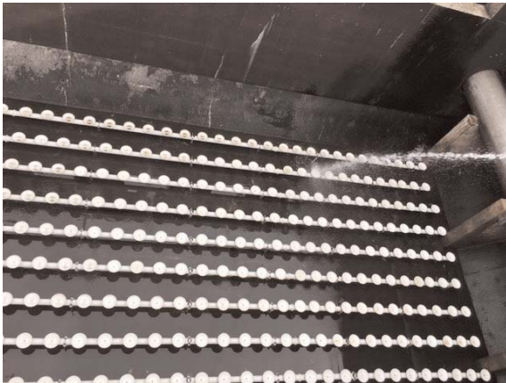
Above: Cleaned and replaced with new membrane diffusers.
