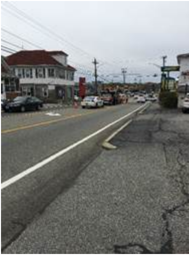
Crew replacing Frame & cover on Mineral Spring Ave.
