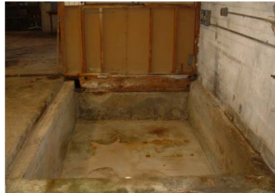
Follow-up inspection of the same facility to verify that the firm has disposed of all solutions and complied with NBC Shutdown Procedures.
