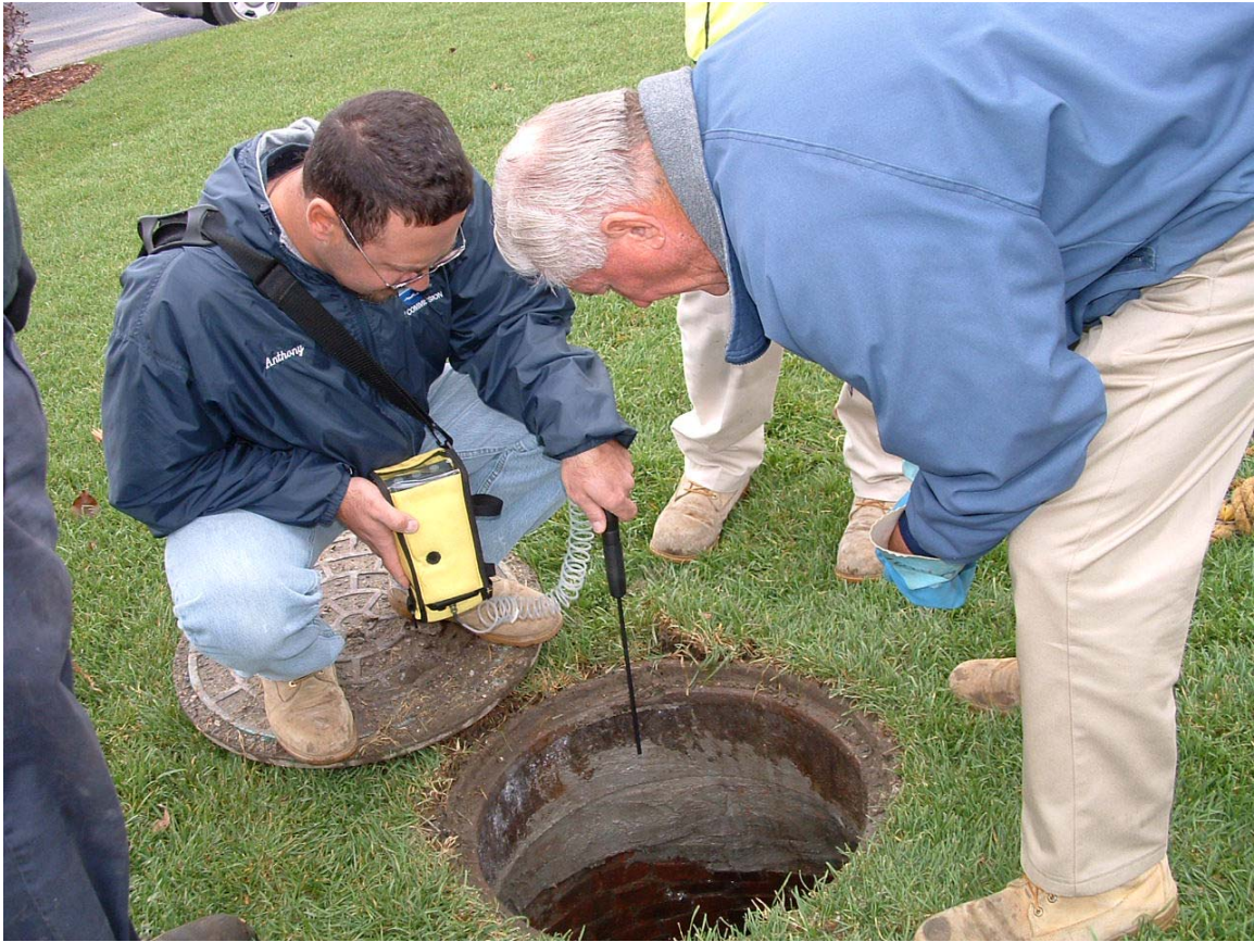
Photo: Manhole inspection
