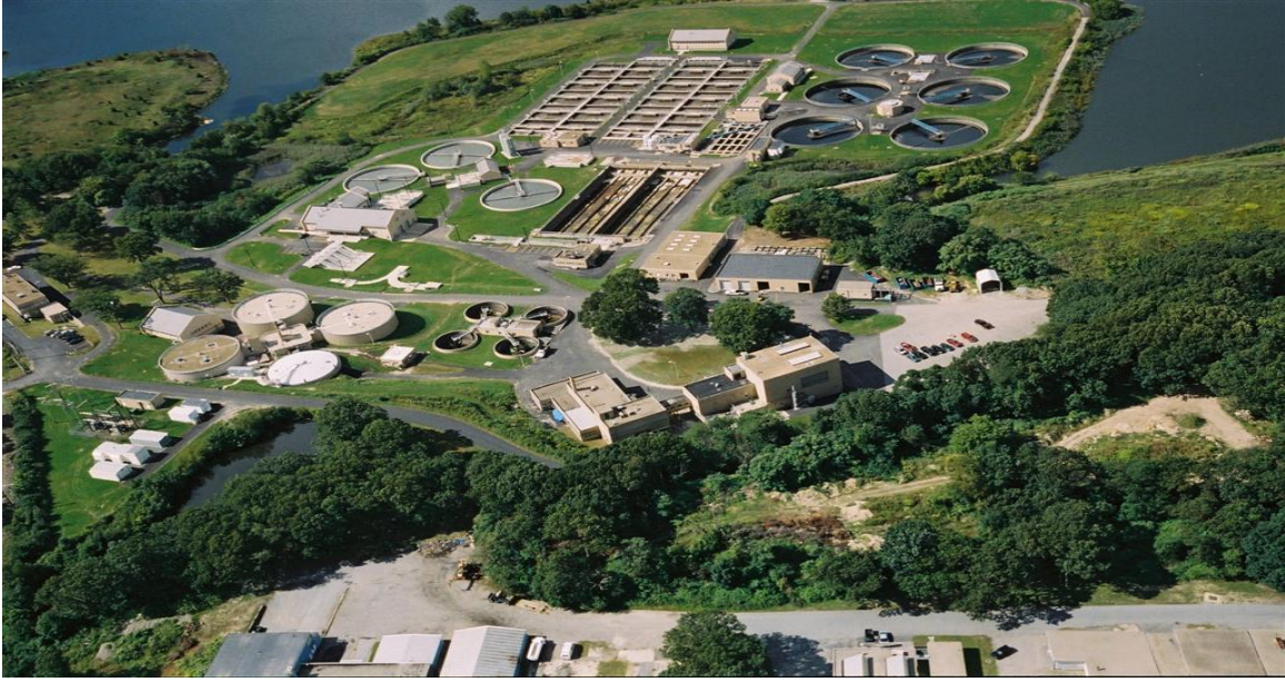
Photo: Bucklin Point Wastewater Treatment Facility
