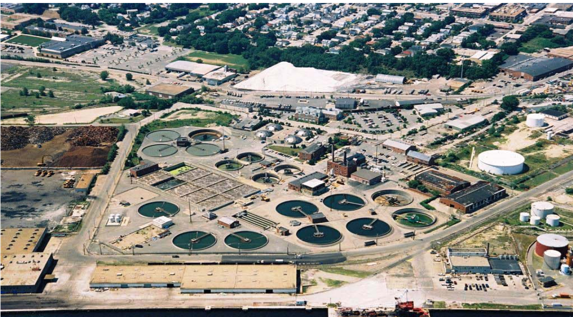
Photo: Field's Point Wastewater Treatment Facility
