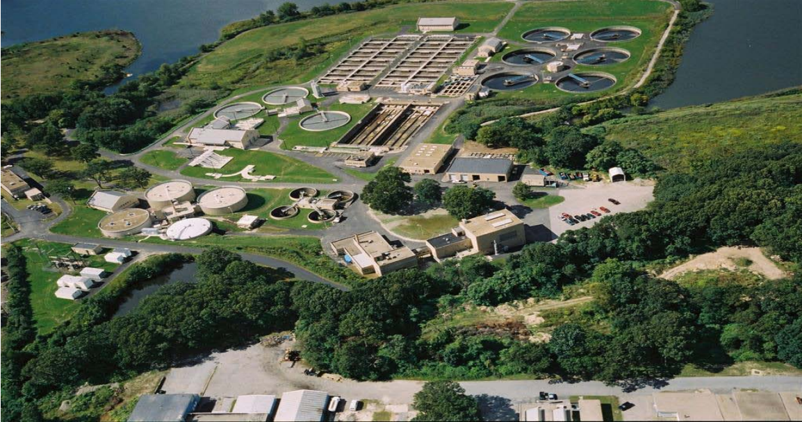
Photo: Bucklin Point Wastewater Treatment Facility
