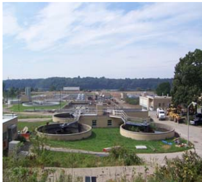
Photo: Bucklin Point Wastewater Treatment Facility.
