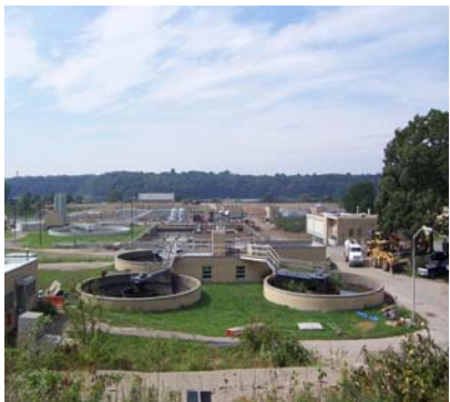
Photo: Bucklin Point Wastewater Treatment Facility.
