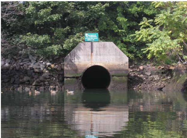
Photo: This combined sewer overflow is located in the Providence River in Providence.
