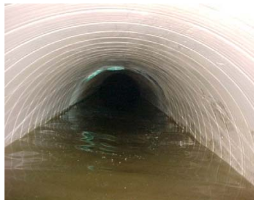
Before and After: The OF 051 emergency repair, located along the Woonasquatucket River, under the Manton Avenue Bridge. The headwall had disintegrated and there were severe voids in the masonry. To repair the pipe, it was lined with Hobas, a glass-fiber reinforced, high-density non-porous liner, which is resilient and abrasion resistant.
