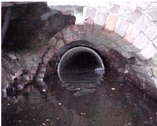
Before and After: The OF 051 emergency repair, located along the Woonasquatucket River, under the Manton Avenue Bridge. The headwall had disintegrated and there were severe voids in the masonry. To repair the pipe, it was lined with Hobas, a glass-fiber reinforced, high-density non-porous liner, which is resilient and abrasion resistant.
