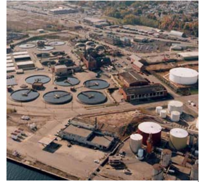
Photo: Aerial photo of the Field's Point Wastewater Treatment Facility
