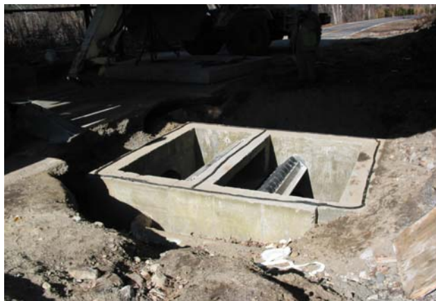
Photo: New diversion structure, awaiting a roof cap
