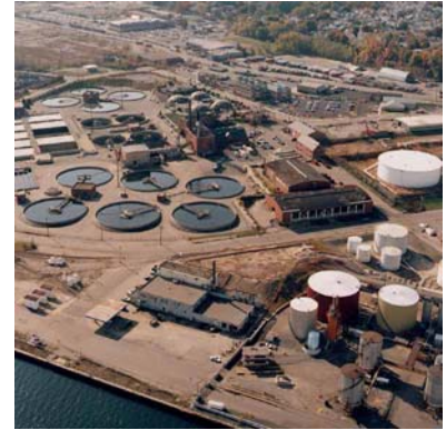
Photo: Aerial photo of the Field's Point Wastewater Treatment Facility
