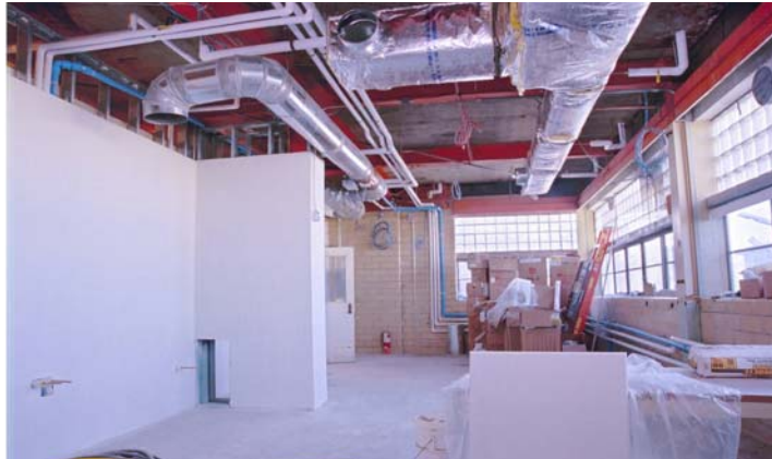
Photo: Bucklin Point Laboratory renovation
