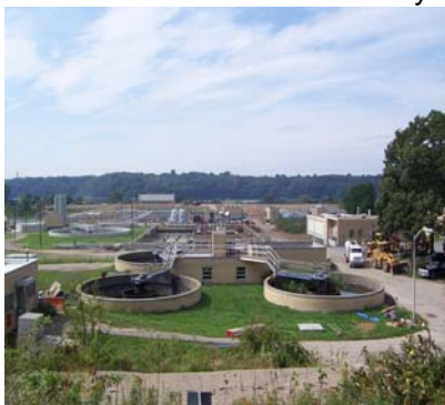
Photo: Bucklin Point Wastewater Treatment Facility.
