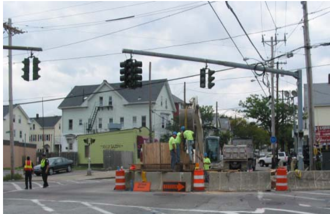
Photo: Police diverting traffic through construction near Atwells Ave.
