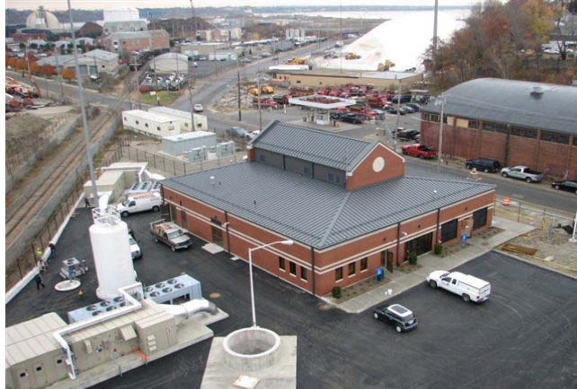
Photo: Tunnel Pump Station, located near Ernest and Ellis Streets
