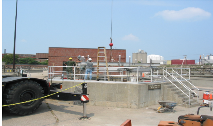
Photo: Replacing of final clarifier splitter box gates, built in the 1980's
