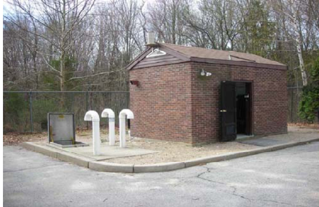
Photo: The Central Avenue Pump Station
