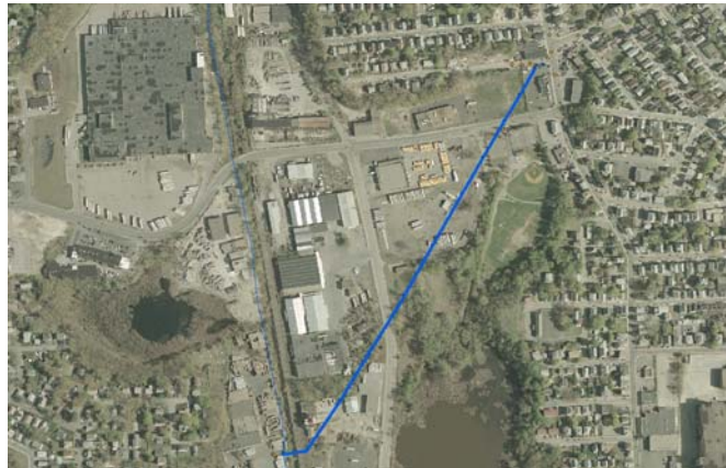
Photo: Portion of the sinking Moshassuck Valley Interceptor
