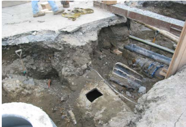
Photo: Removal of abandoned pipe at Atwells Ave. and Valley Street
