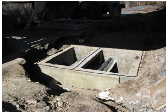
Photo: New diversion structure, awaiting a roof cap
