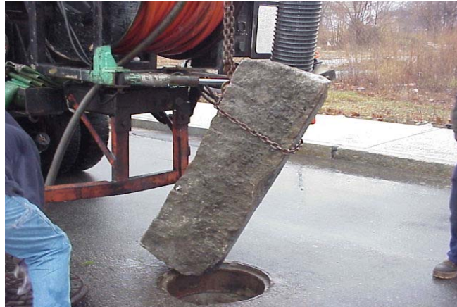
Photo: Granite curbing removal from Ocean Street Interceptor
