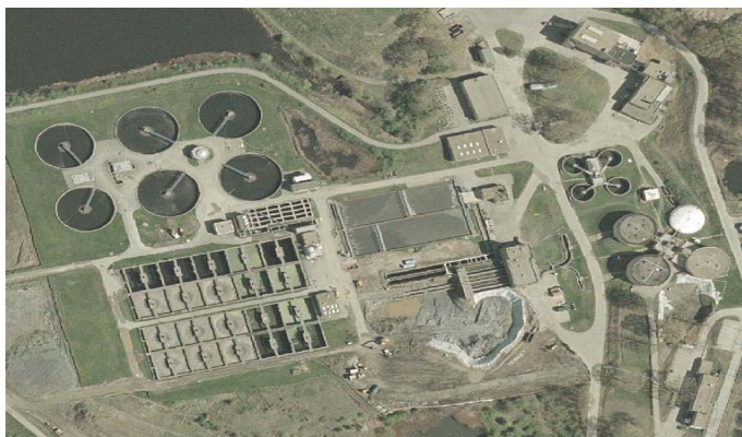
Photo: Aerial view of the BPWWTF
