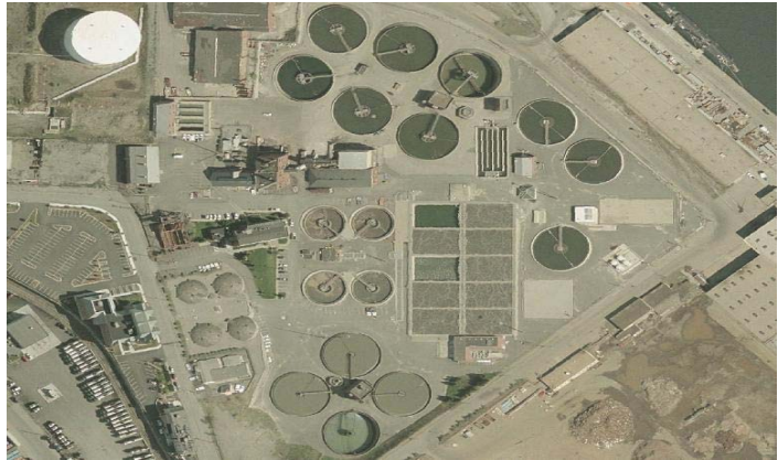
Photo: Aerial view of the FPWWTF
