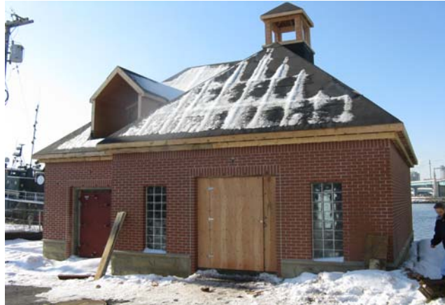
Photo: The Siphon Gate House
