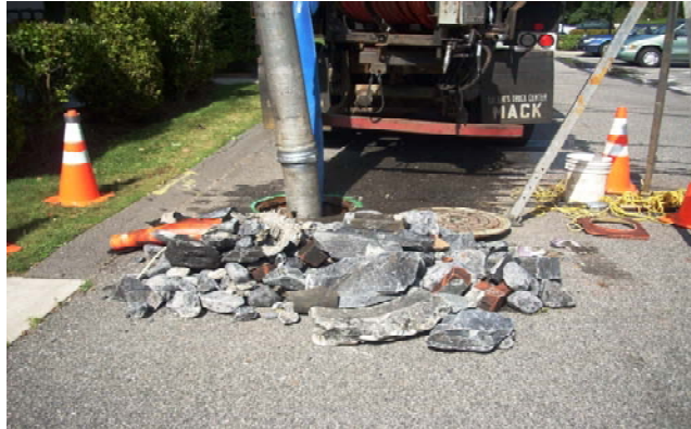
Photo: Heavy rock debris removed from sewer off Manton Ave
