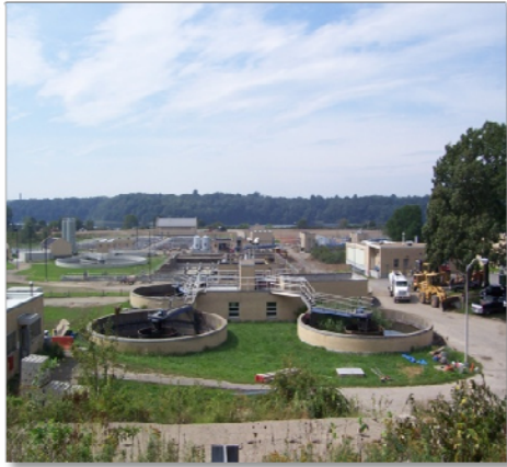
Photo: Bucklin Point Wastewater Treatment Facility
