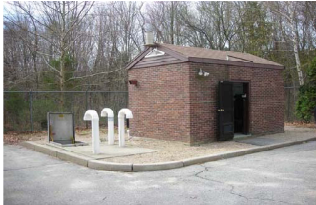
Photo: The Central Avenue Pump Station
