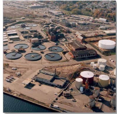
Photo: Aerial View of Field's Point
