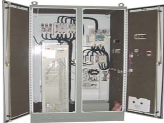
Photo: A schematic of a variable frequency drive unit
