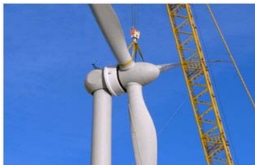
Photo: Assembly of a pre-built wind turbine
