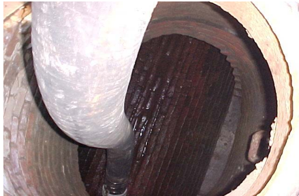
Photo: Bypass Pumping brick sewer prior to pipe lining
