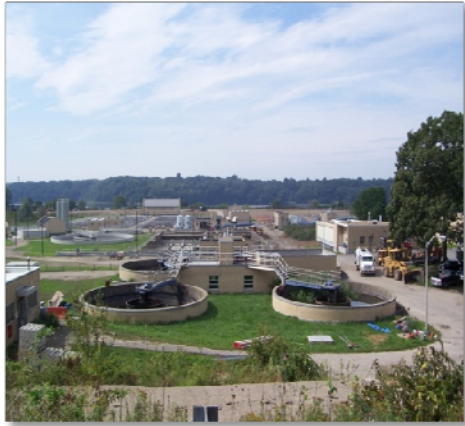
Photo: Bucklin Point Wastewater Treatment Facility
