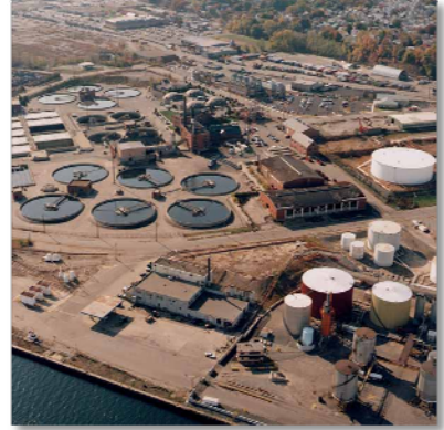
Photo: Aerial View of Field's Point
