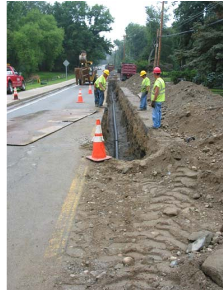
Above: An improvement project near Central Avenue.
