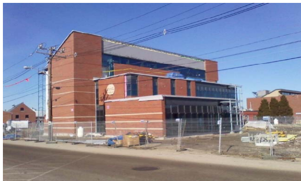
Photo: Newly constructed Operations building.
