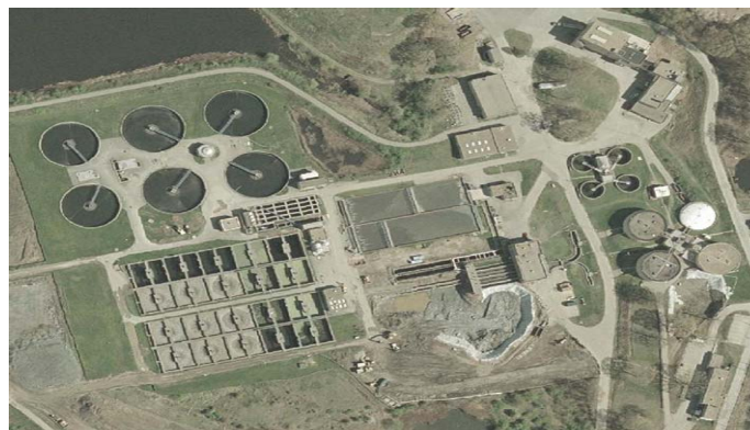
Photo: Aerial view of the BPWWTF
