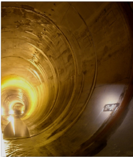
Photo: A view of a portion of the completed three mile long CSO Tunnel
