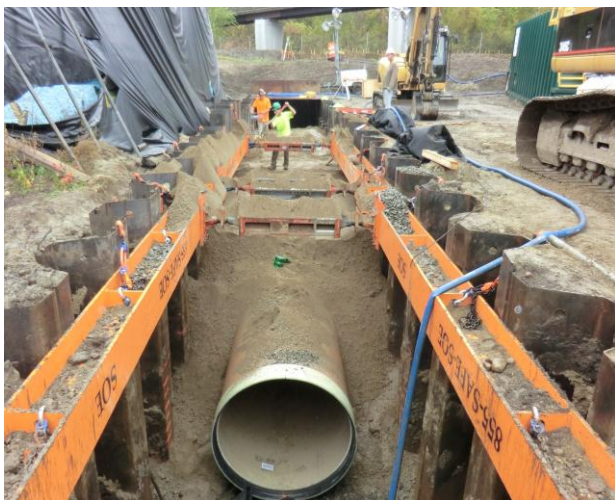
Photo: Woonasquatucket CSO Interceptor West - Piping Installation
