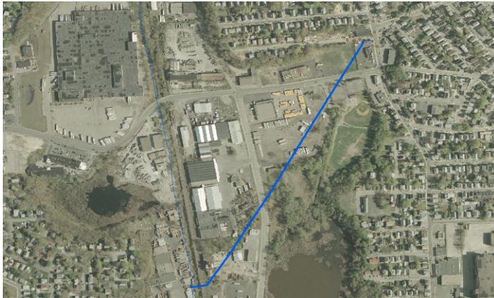
Photo: Portion of the Mosshassuck Valley Interceptor to be replaced Project Overview
