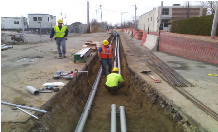
Photo: Utility work being performed on Service Road Project Overview
