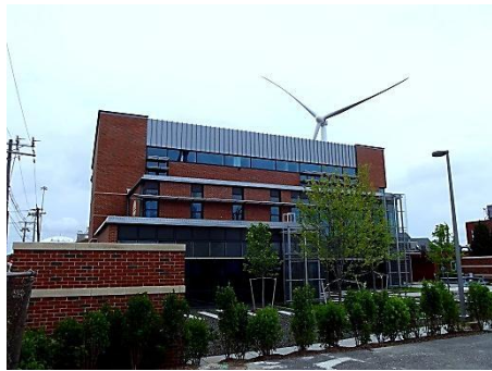
Photo: New Operations Building - Field's Point
