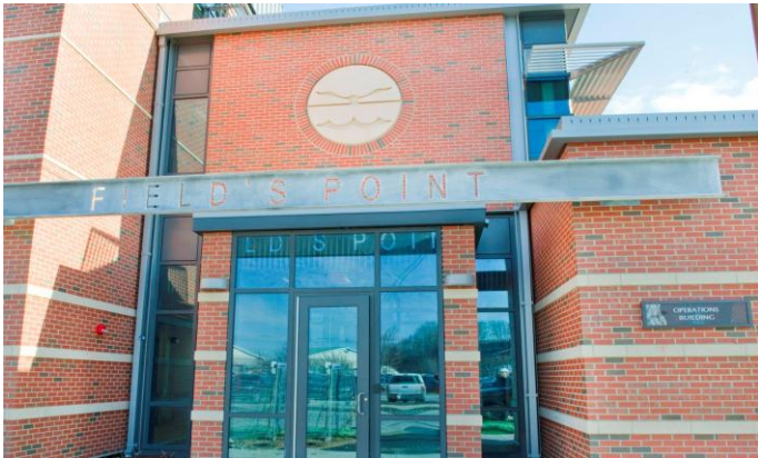
Photo: Newly constructed Operations Building Project Overview
