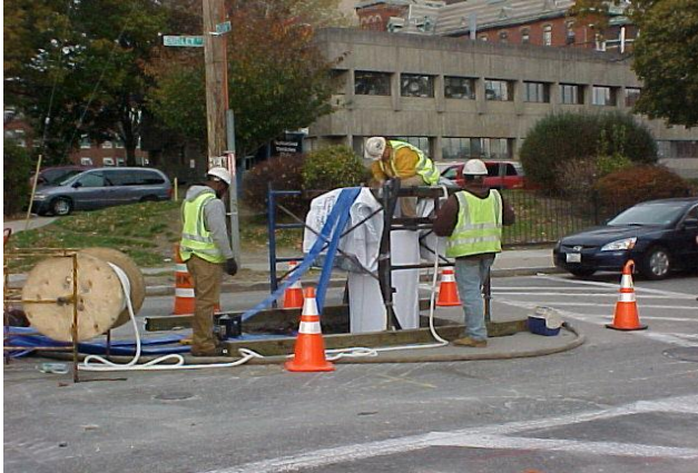
Photo: Lining at an interceptor improvement location Project Overview
