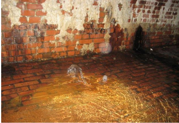
Photo: Infiltration into existing WCSOI North overflow Project Overview
