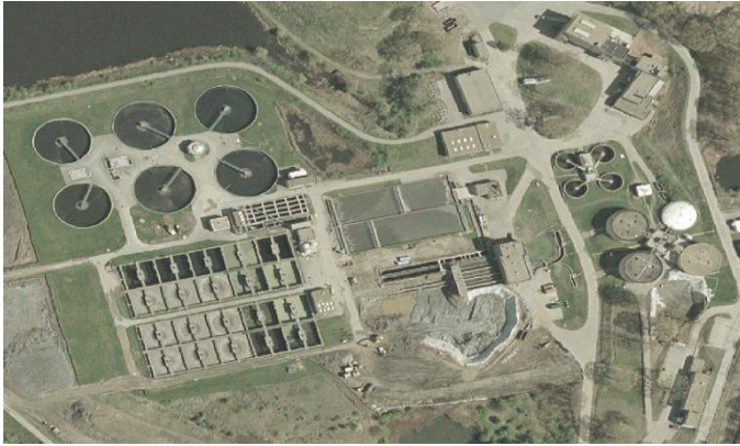
Photo: Aerial view of the BPWWTF Project Overview
