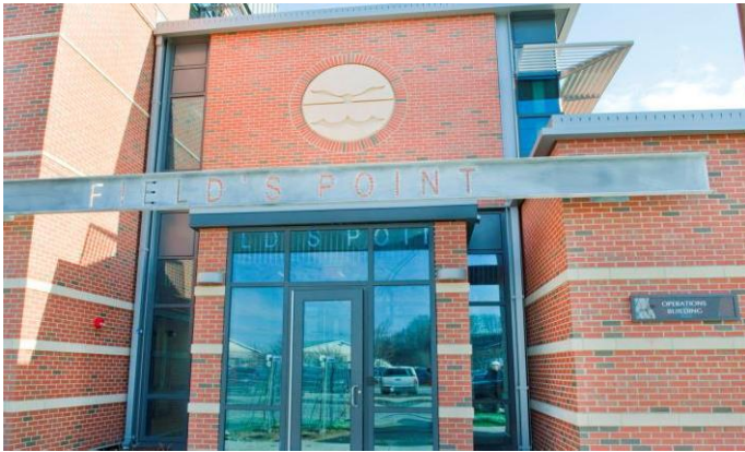
Photo: Newly constructed Operations Building Project Overview
