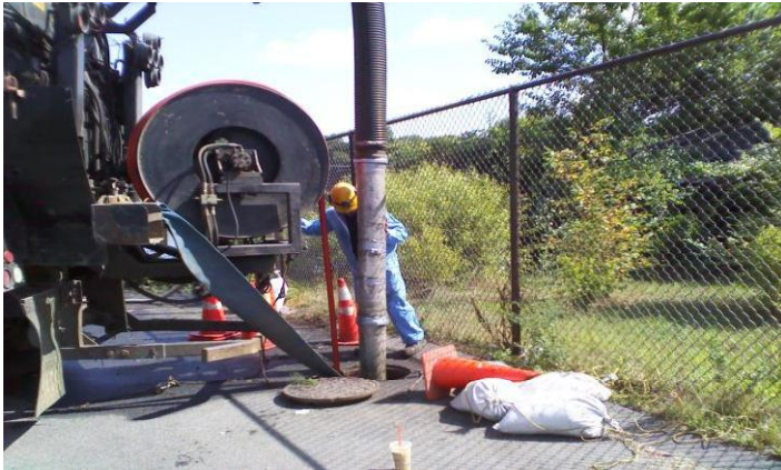
Photo: Cleaning the sewer at the Omega Pump Station Project Overview
