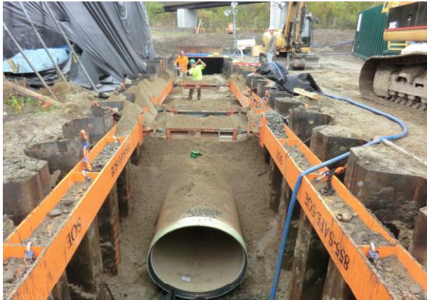
Photo: Piping Installation north of Route 6 in Johnston Project Overview
