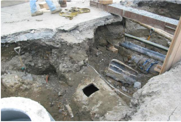
Photo: Removal of abandoned pipe at Atwells Ave. and Valley Street Project Overview
