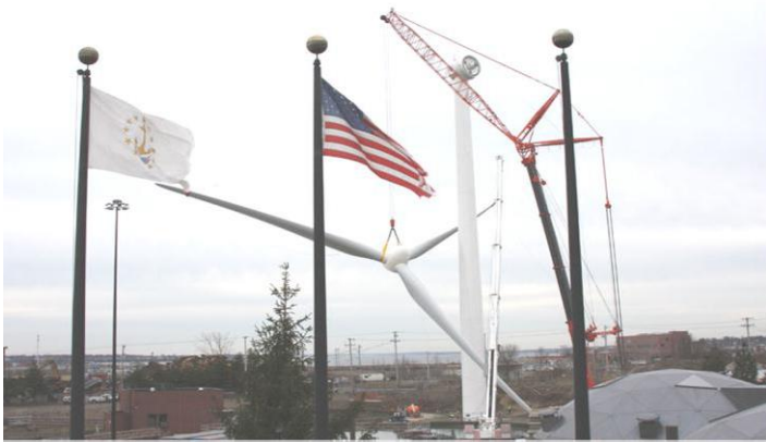
Photo: The blades being connected to the hub Project Overview
