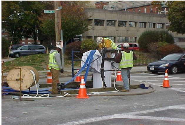
Photo: Working at an interceptor improvement location Project Overview
