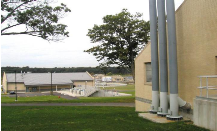
Photo: Bucelin Point Boiler Plant
