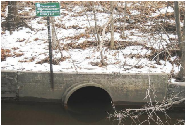
Photo: CSO 017 at Cemetery Street Project Overview
