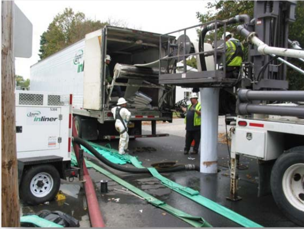
Photo: Inverting of lining at an interceptor improvement location
