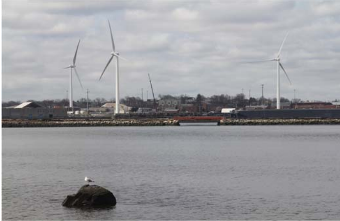
Photo: Field's Point Wind Turbines
