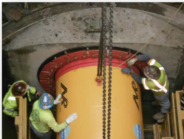
Photo: Woonasquatucket CSO Interceptor - Piping Installation
