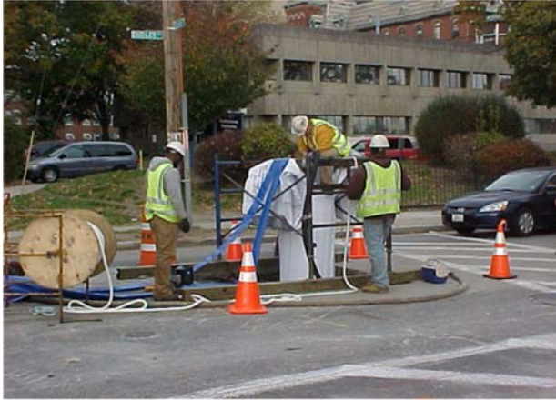
Photo: Lining at an interceptor improvement location
