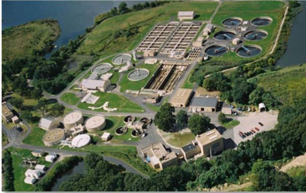
Photo: Bucklin Point Wastewater Treatment Facility
