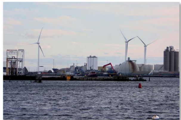
Photo: Field’s Point Wind Turbines
