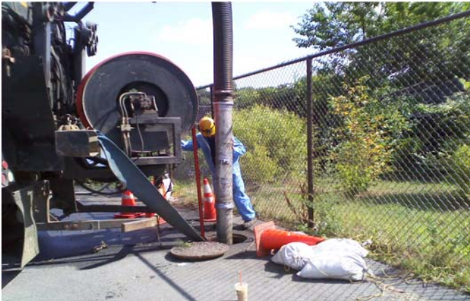
Photo: Cleaning the sewer at the Omega Pump Station
