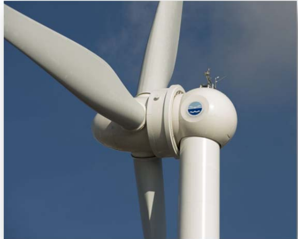
Photo: One of three wind turbines at Fields Point
