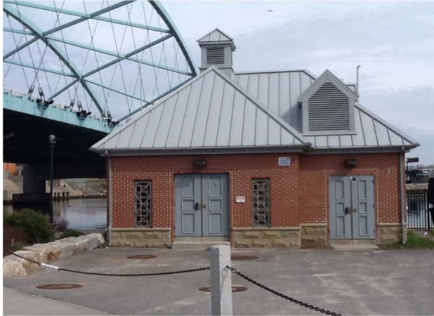
Photo: Providence River Siphon House
