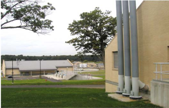
Photo: Bucklin Point Boiler Stacks
