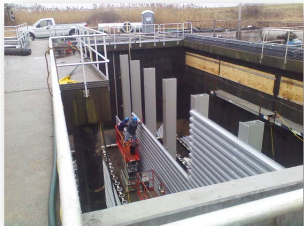
Photo: Reconfiguring of aeration tank at Bucklin Point
