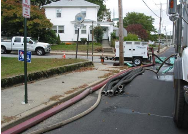
Photo: Lining at an interceptor improvement location
