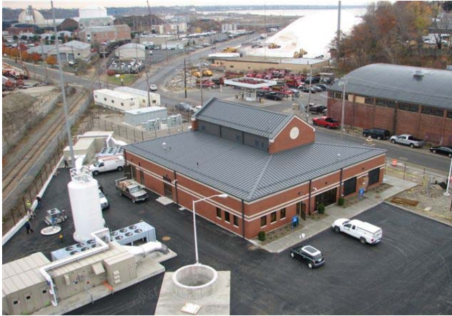
Photo: Tunnel Pump Station
