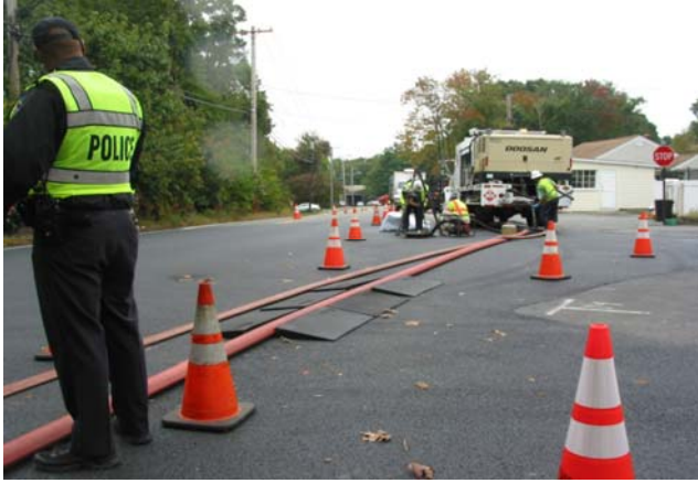
Photo: Lining at an interceptor improvement location
