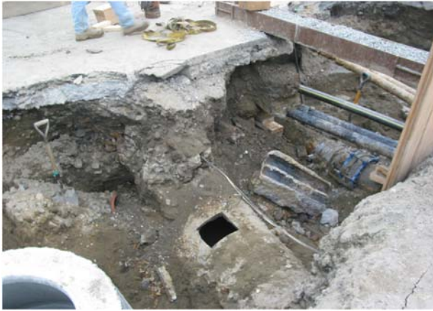
Photo: Removal of abandoned pipe at Atwells Ave. and Valley Street
