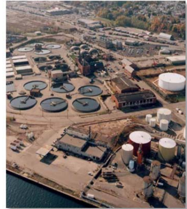
Photo: Aerial View of Field's Point
