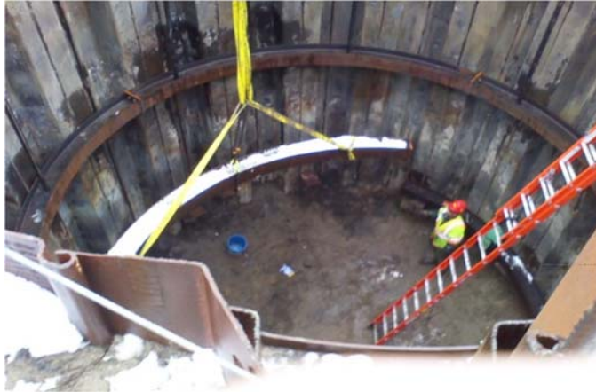
Photo: Installation of waler supports
