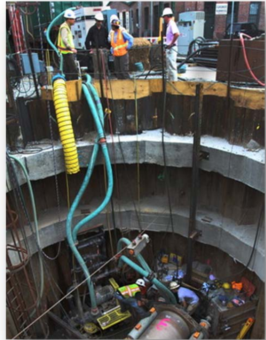
Photo: Tunneling pipe for the Woonasquatucket Interceptor
