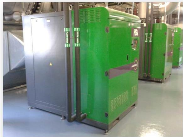
Photo: New turbo blowers at Field's Point
