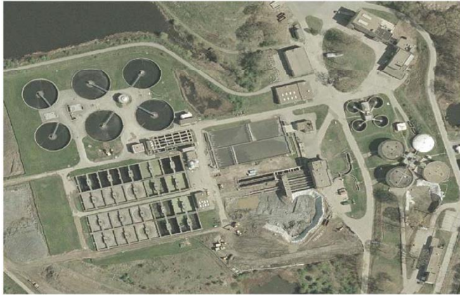
Photo: Aerial view of the BPWWTF Project Overview
