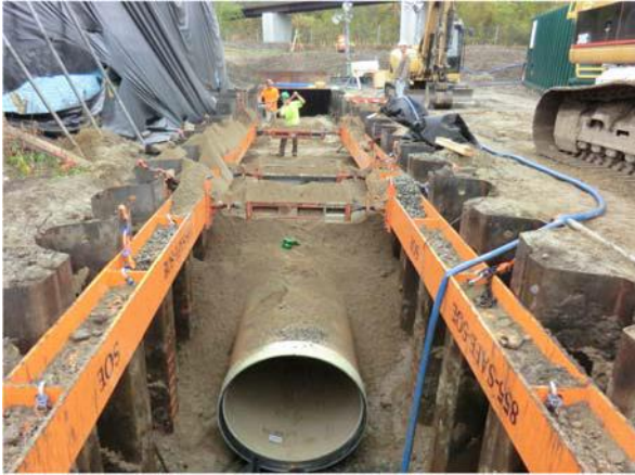
Photo: Piping Installation north of Route 6 in Johnston
