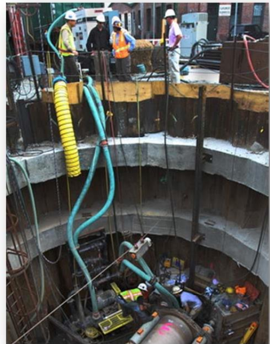
Photo: Tunneling pipe for the Woonasquatucket Interceptor
