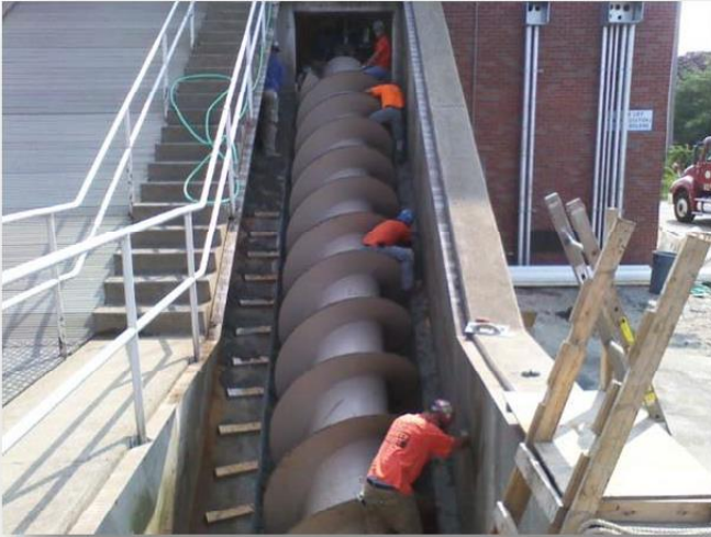
Photo: Workers placing grout for replaced screw lift pumps
