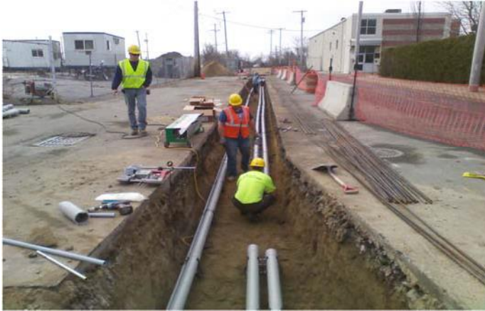
Photo: Utility work being performed on Service Road
