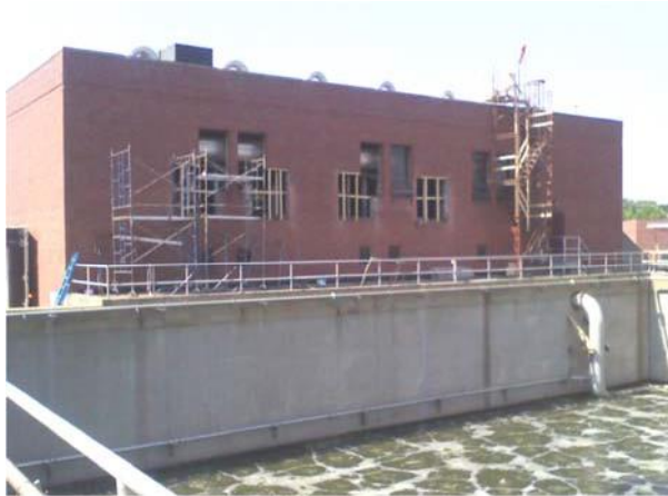
Photo: Blower Building Louver Cut-outs
