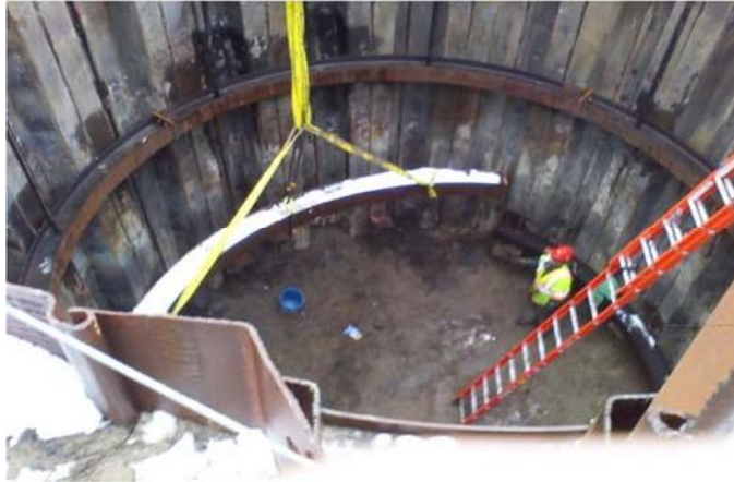
Photo: Installation of water supports Project Overview
