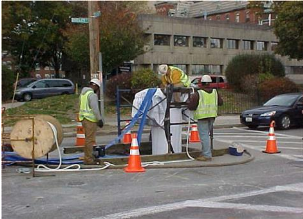
Photo: Lining at an interceptor improvement location
