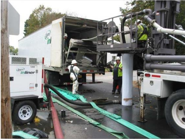
Photo: Inserting of lining at an interceptor in project location
