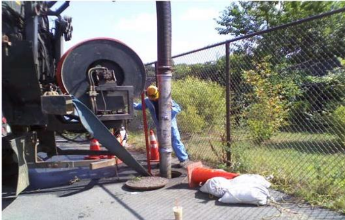
Photo: Cleaning the sewer at the Omega Pump Station Project Overview
