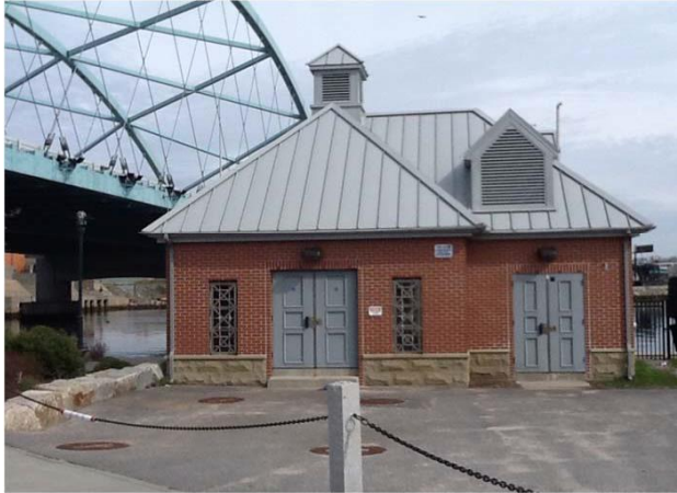
Photo: Providence River Siphon House
