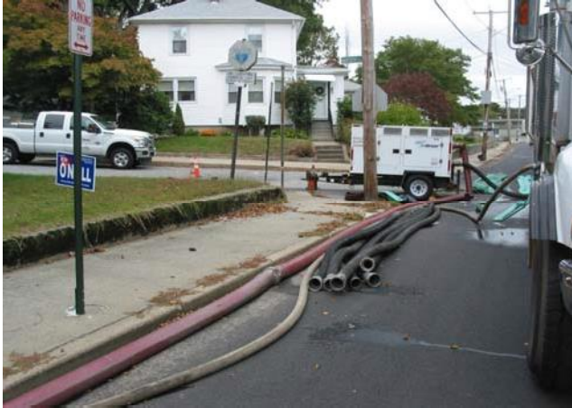
Photo: Lining at an interceptor improvement location
