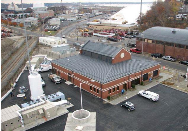
Photo: Tunnel Pump Station
