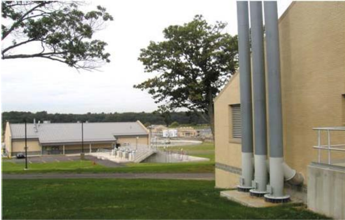
Photo: Bucelin Point Boiler Plant
