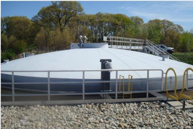
Photo: Digester tank at Bucklin Point
