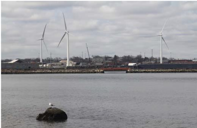
Photo: Field's Point Wind Turbines
