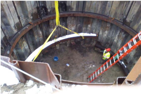
Photo: Installation of waler supports
