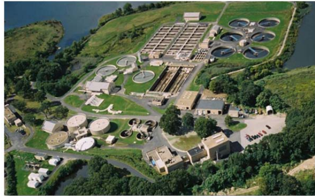
Photo: Bucklin Point Wastewater Treatment Facility
