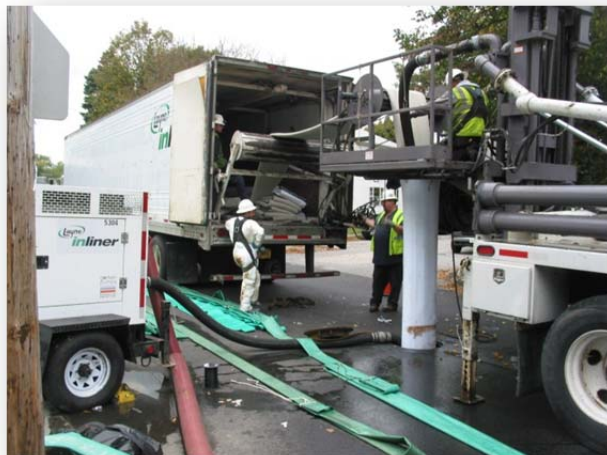
Photo: Inverting of interceptor lining
