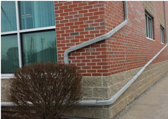
Photo: Downspouts at NBC COB
