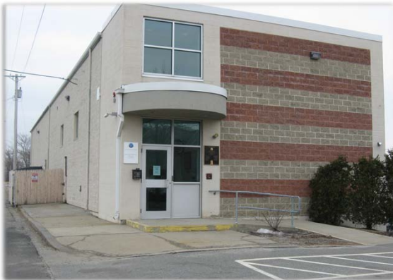
Photo: Existing Lab Building at FPWWTF
