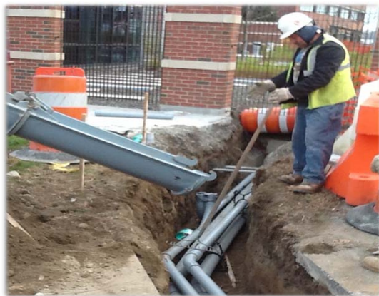
Photo: Utility work being performed on Service Road
