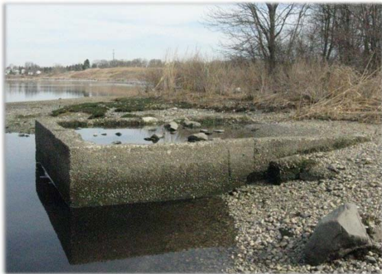
Photo: BPWWTF Outfall
