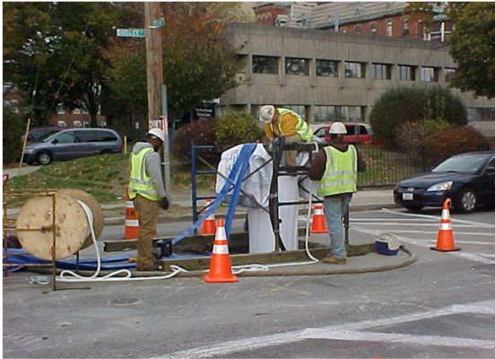
Photo: Lining at an interceptor improvement location
