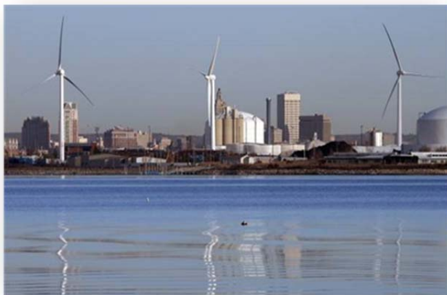
Photo: Field's Point Wind Turbines
