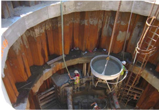
Photo: Tunneling pipe for the Woonasquatucket Interceptor
