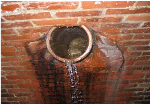
Photo: Infiltration into existing WCSOI North overflow
