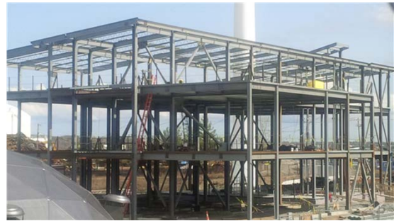
Photo: Steel Construction at the Regulatory Compliance Building
