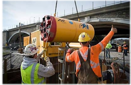
Photo: Digging on East Side of Providence
