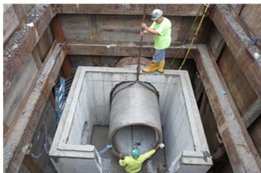
Photo: Seekonk Interceptor Installation
