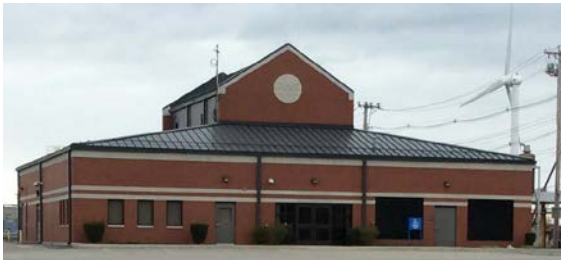
Photo: Tunnel Pump Station
