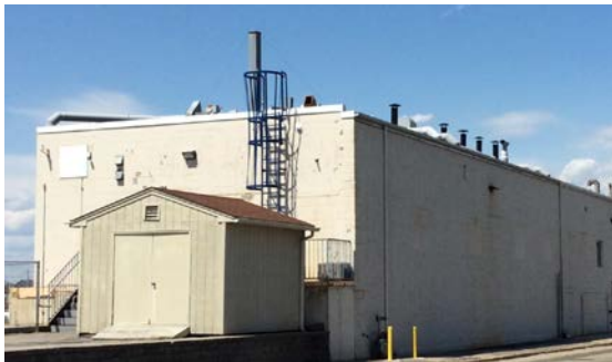
Photo: Existing Laboratory Building
