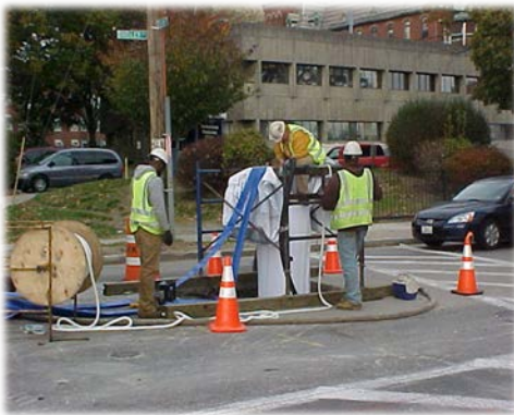
Photo: Lining at an interceptor improvement location
