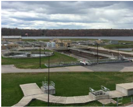
Photo: Bucklin Point WWTF
