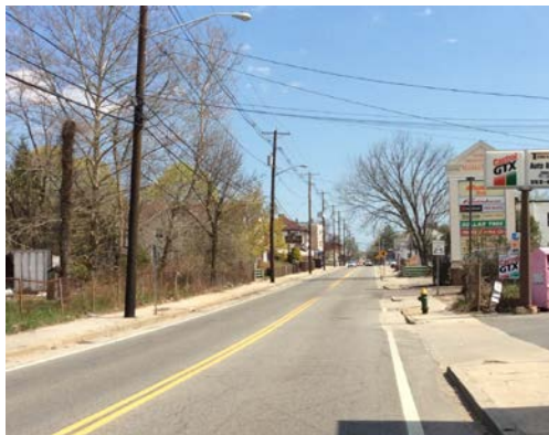
Photo: Branch Avenue Interceptor improvement location
