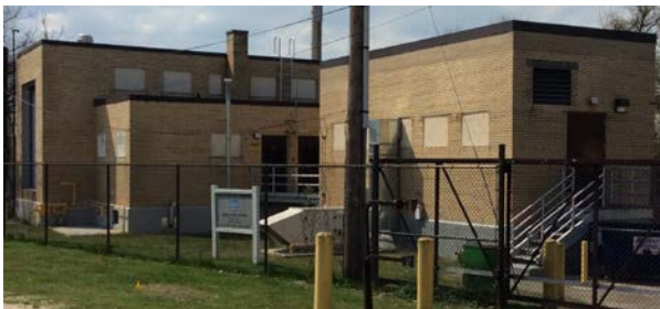
Photo: Omega Pumping Station
