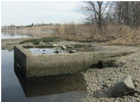
Photo: Bucklin Point WWTF Outfall
