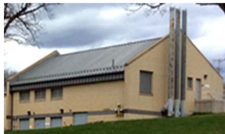
Photo: Bucklin Point Digester building
