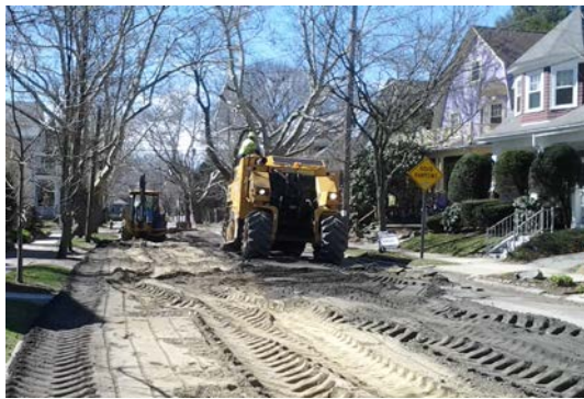
Photo: Fourth Street OF 037 South Sewer Separation location
