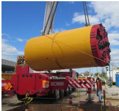
Photo: Micro Tunnel Boring Machine Installation
