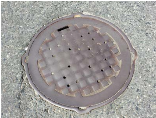
Photo: Municipal Sewer Manhole Cover
