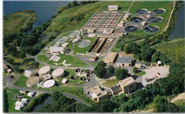
Photo: Bucklin Point Wastewater Treatment Facility
