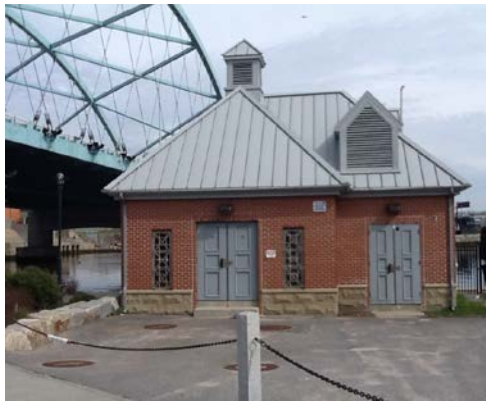
Photo: Providence River Siphon House
