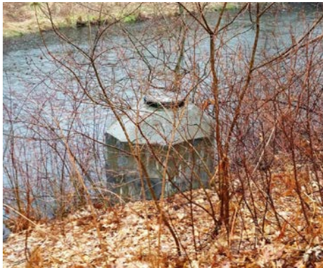
Photo: Manhole along river
