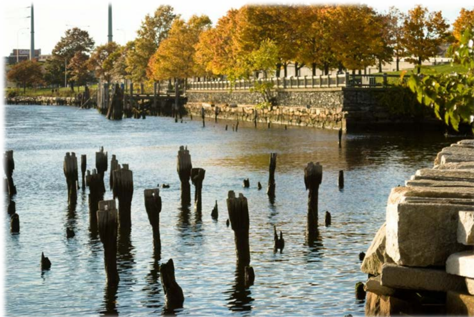
Photo: Old Pier Piles at India Point Park, Seekonk River
