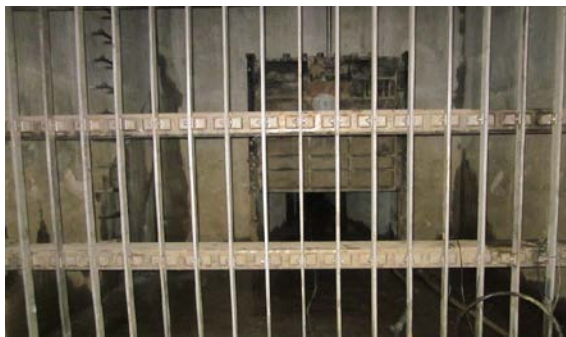
Photo: Bar Screens in Gate and Screening Structure
