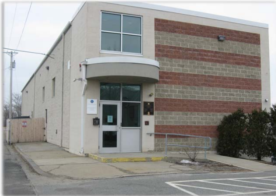
Photo: Existing Lab Building at FPWWTF
