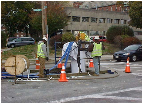
Photo: Lining at an interceptor improvement location
