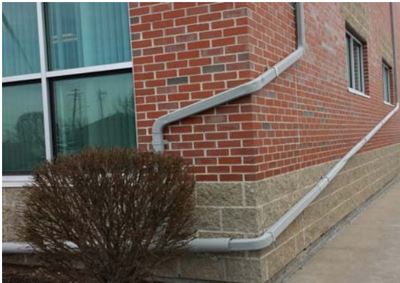
Photo: Downspouts at NBC COB
