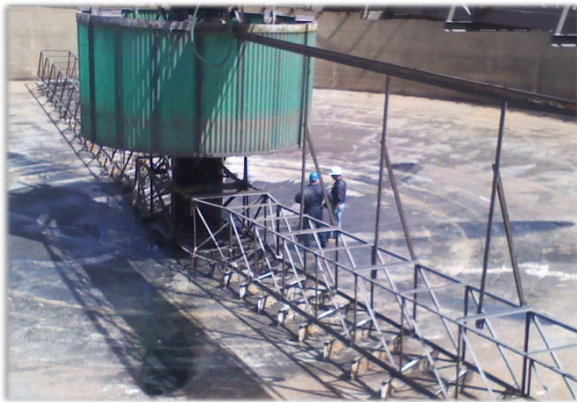
Photo: Inspecting Primary Clairifiers
