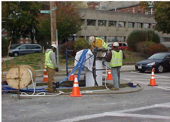
Photo: Lining at an interceptor improvement location
