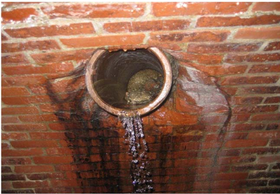
Photo: Infiltration into existing WCSOI North overflow
