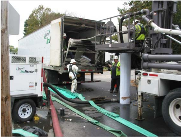
Photo: Inverting of interceptor lining
