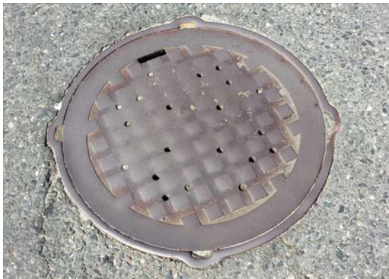
Photo: Municipal Sewer Manhole Cover
