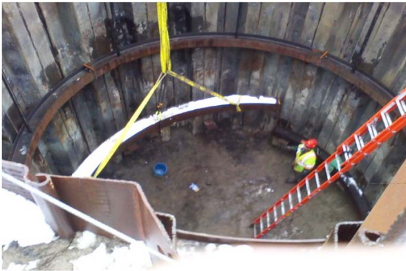
Photo: Installation of waler supports
