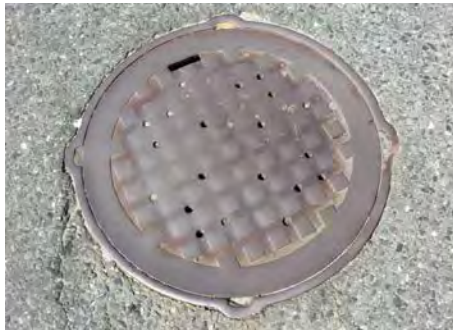
Photo: Municipal Sewer Manhole Cover
