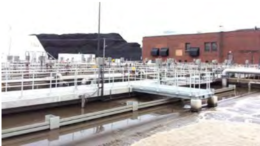
Photo: Aeration tanks at Field's Point
