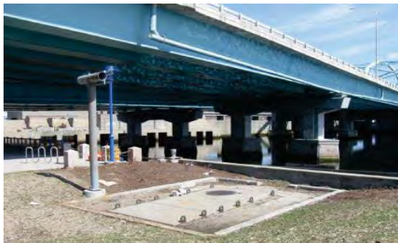
Photo: Siphon Trail Chamber
