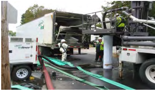
Photo: Conducting Sewer System Repairs
