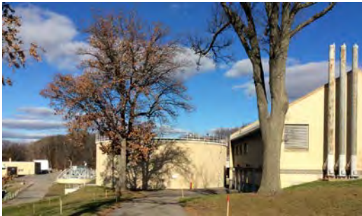
Photo: Bucklin Point Boiler Stacks
