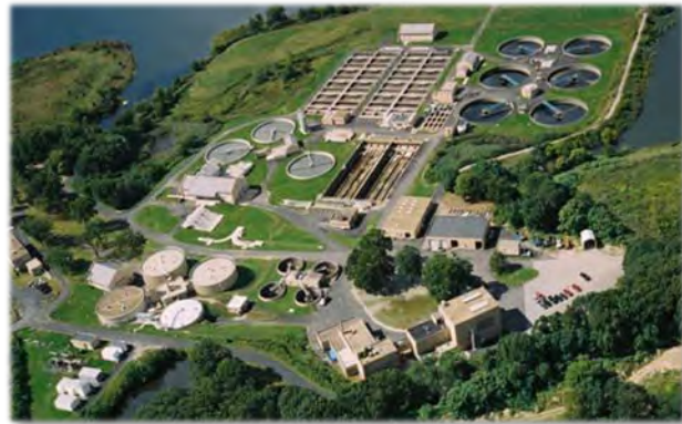
Photo: Bucklin Point Wastewater Treatment Facility
