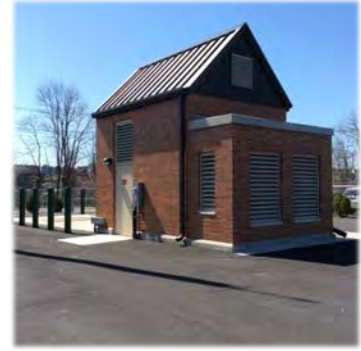
Photo: WCS01 Gate & Screening Structure
