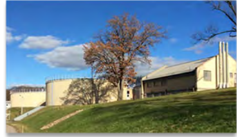
Photo: Bucklin Point Digester Building
