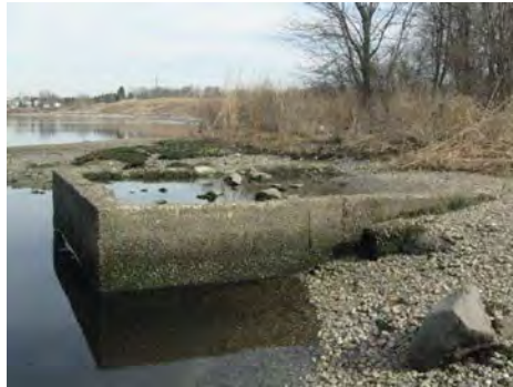
Photo: Bucklin Point WWTF Outfall
