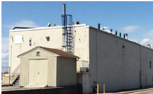
Photo: Existing Laboratory Building
