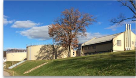
Photo: Bucklin Point Digester Building
