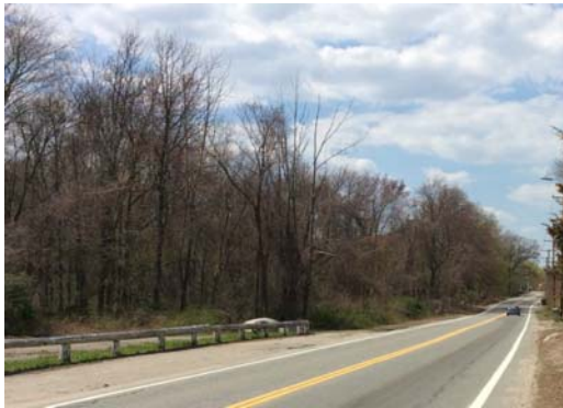
Photo: Lincoln Interceptor Replacement Location
