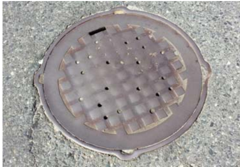
Photo: Municipal Sewer Manhole Cover
