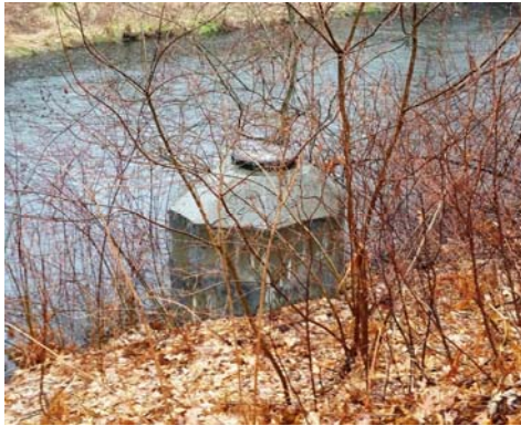
Photo: Manhole along river
