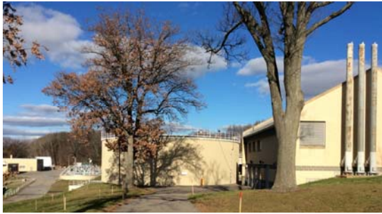
Photo: Bucklin Point Boiler Stacks
