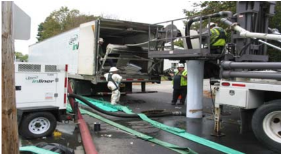
Photo: Conducting Sewer System Repairs
