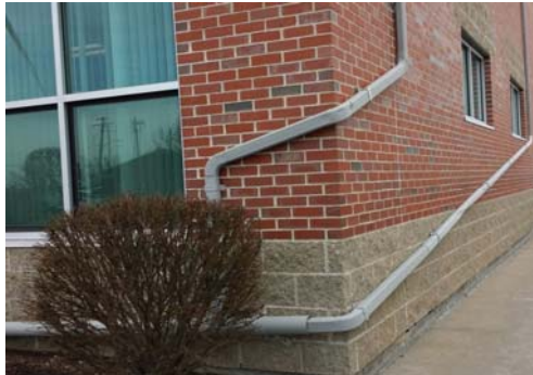
Photo: Downspouts at the NBC COB
