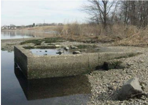
Photo: Bucklin Point WWTF Outfall
