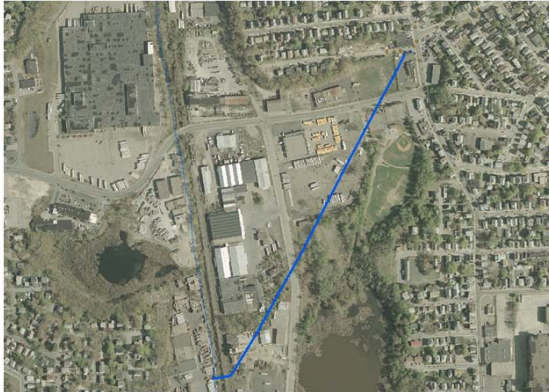
Photo: Portion of the Mosshassuck Valley Interceptor to be replaced
