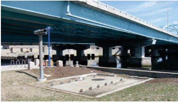
Photo: Siphon Trail Chamber
