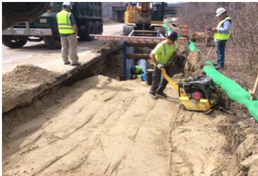
Photo: Construction on Greenville Avenue
