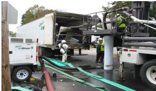
Photo: Conducting Sewer System Repairs
