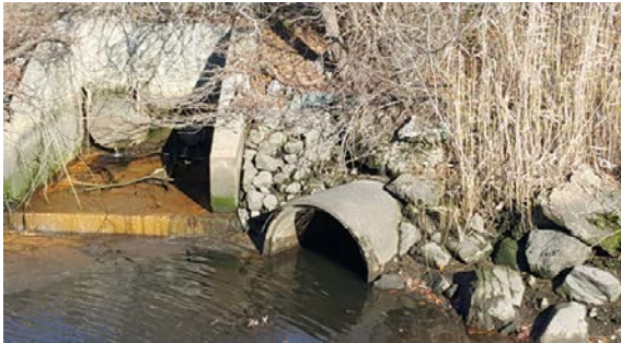
Photo: End of North Outfall Pipe
