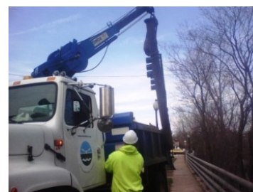
Photo: Removing Catch Basin Sediment
