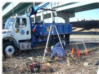
Photo: NBC's staff utilizing a digger
