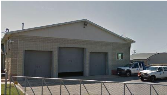
Photo: Existing IM Building
