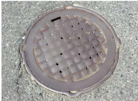
Photo: Municipal Sewer Manhole Cover
