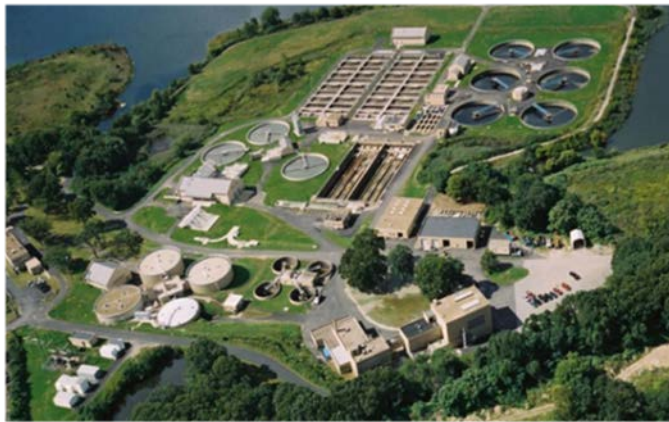
Photo: Bucklin Point Wastewater Treatment Facility
