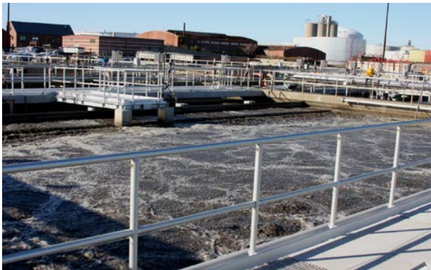
Photo: Aeration Tanks FPWWTF
