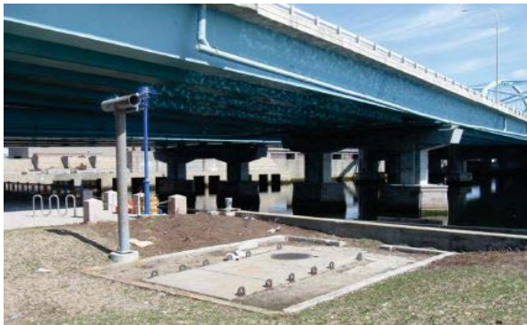
Photo: Siphon Outlet Chamber
