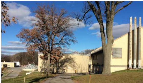
Photo: Bucklin Point Digester and Heat Exchanger Building
