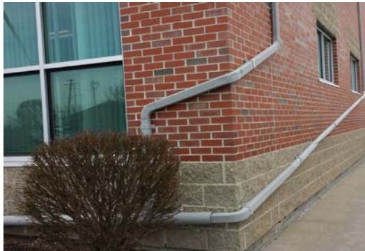
Photo: Downspouts at the NBC COB
