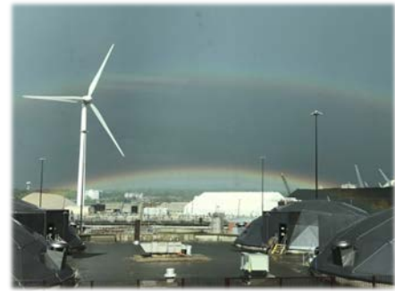
Photo: Field's Point Wind Turbine
