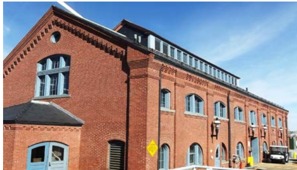
Photo: Existing Maintenance Building
