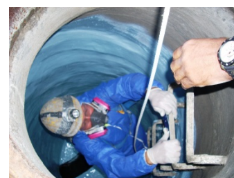
Photo: Interceptor Inspection
