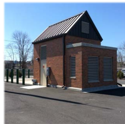
Photo: WCS01 Gate & Screening Structure
