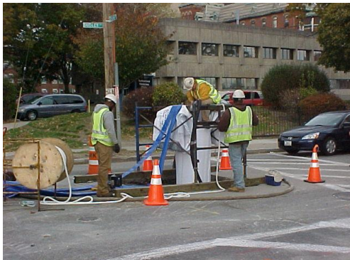
Photo: Conducting Sewer System Repairs
