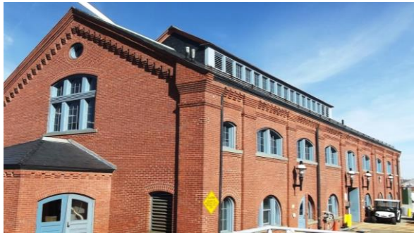
Photo: Existing Maintenance Building
