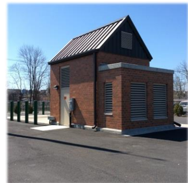
Photo: WCS01 Gate & Screening Structure
