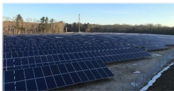
Photo: Solar Array in Richmond, RI
