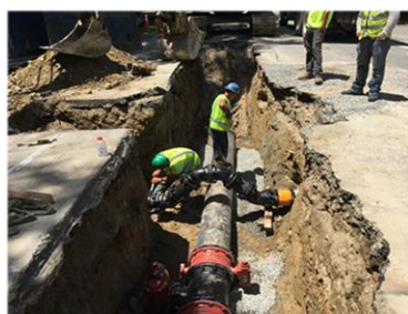
Photo: Interceptor Installation in Johnston
