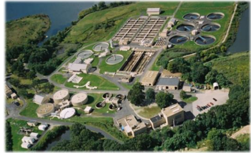
Photo: Bucklin Point Wastewater Treatment Facility
