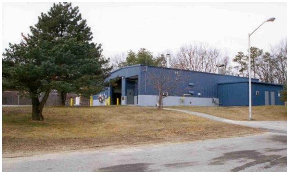
Photo: Septage Receiving Station
