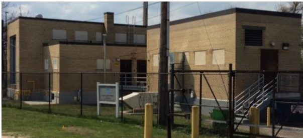
Photo: Omega Pump Station
