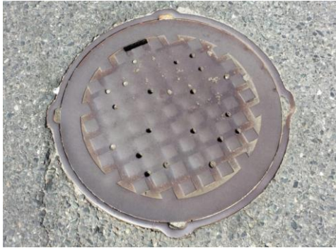
Photo: Municipal Sewer Manhole Cover
