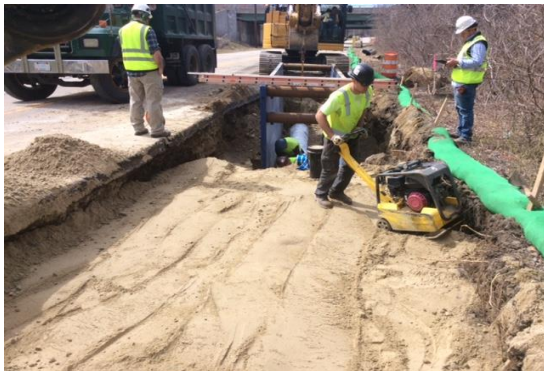
Photo: Construction on Greenville Avenue
