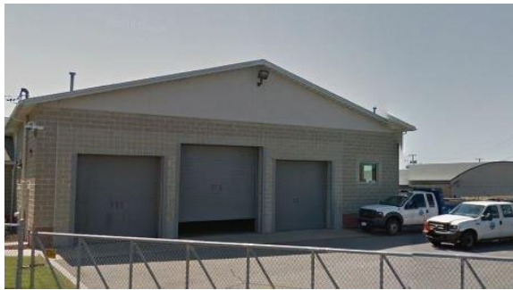
Photo: Existing IM Building
