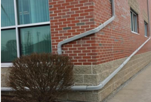
Photo: Downspouts at NBC's Corporate Office Building
