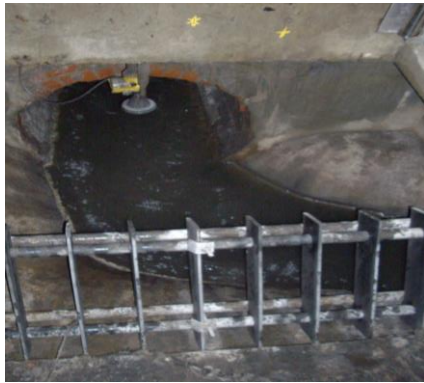
Photo: Flow Meter Installed
