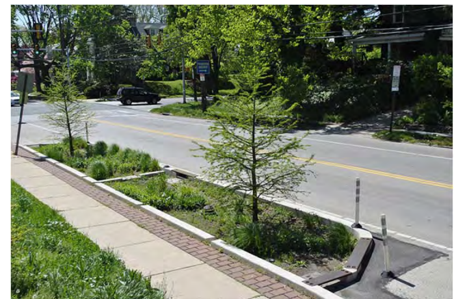
Corner Stormwater Bump-out
