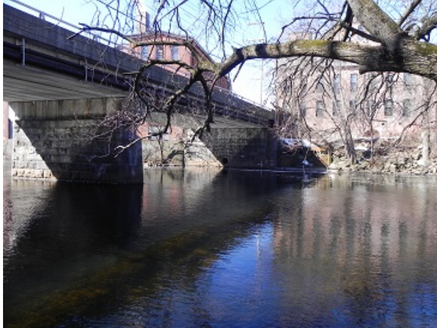
Figure 4-34 - Cross St Bridge
