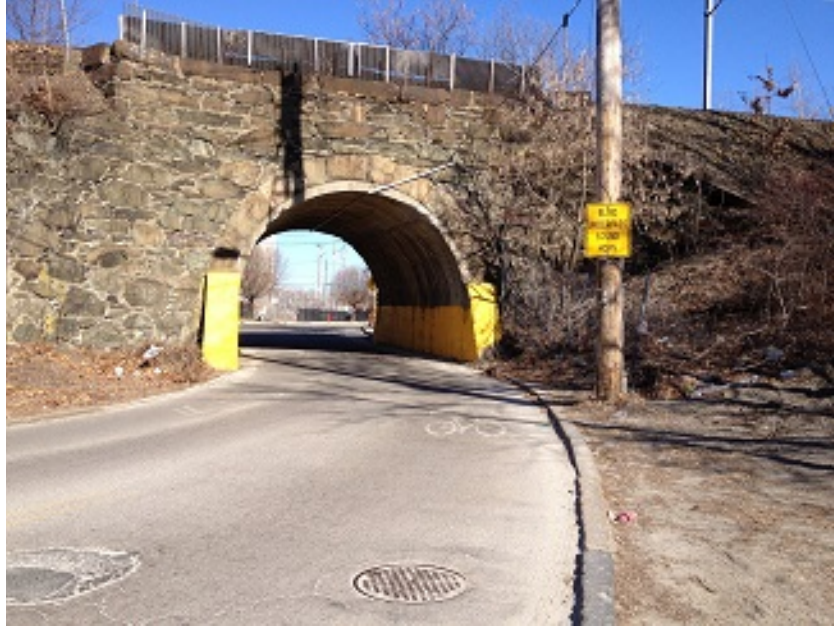
Figure 4-33 - High St Railroad Overpass
