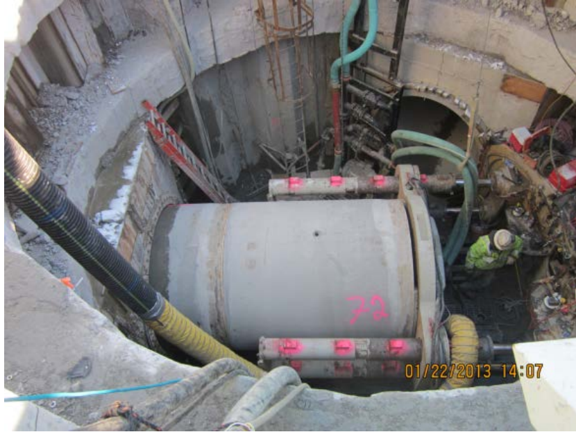
Figure 4-26 – NBC Phase II Interceptor Construction
