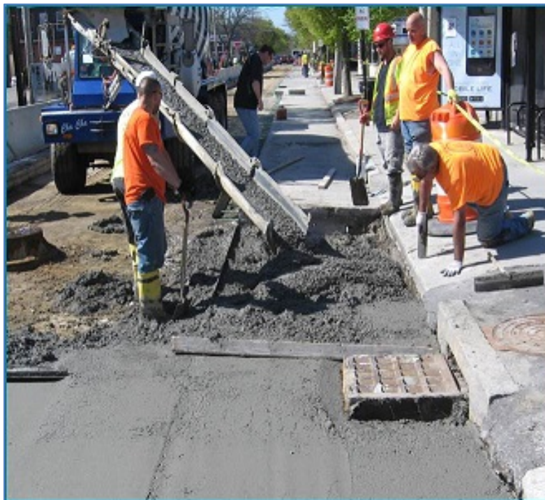
Figure 4-8 - NBC Phase 2 Sewer Separation Surface Restoration
