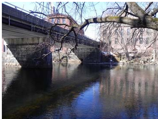
Figure 45 - Cross St Bridge
