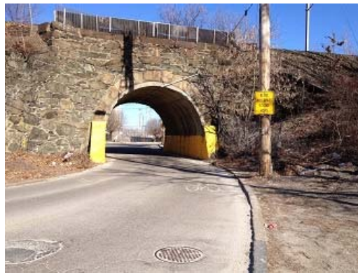
Figure 44 - High St Railroad Overpass
