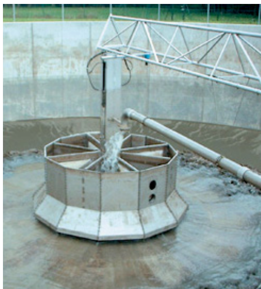
Figure 57 – Example of Round Tank Flushing System
