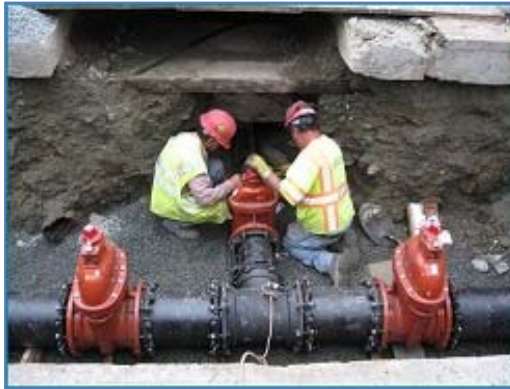
Figure 18 - NBC Phase II Sewer Separation Utility Installation
