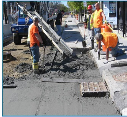
Figure 20 - NBC Phase 2 Sewer Separation Surface Restoration
