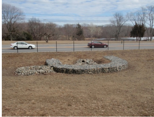
Figure 4 - Stormwater Flow Control - Detention Storage
