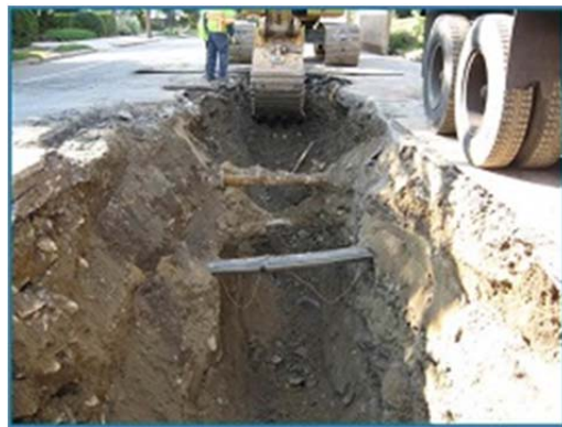
Figure 19 - NBC Phase II Sewer Separation Utility Conflicts
