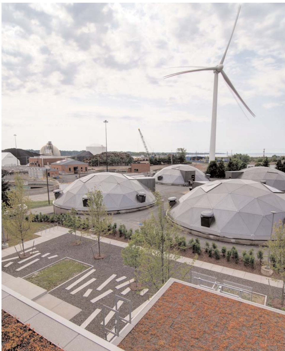
A view of the green roof, native plantings, and reused concrete and asphalt from the Commission's new Silver LEED Designed Administration Building at the Field's Point Wastewater Treatment Facility. One of the Commission's three 1.5 mW wind turbines is in the background.
