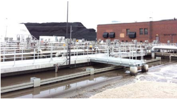
Photo: Field's Point Aeration Treatment Process
