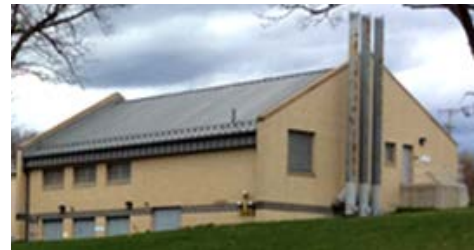
Photo: Bucklin Point Digester building
