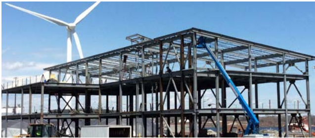
Photo: Regulatory Compliance Building Steel Framing
