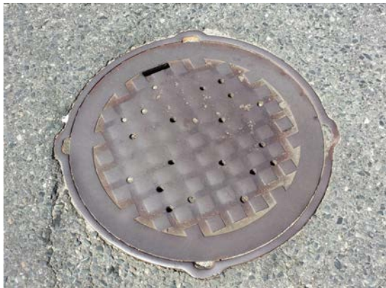
Photo: Municipal Sewer Manhole Cover
