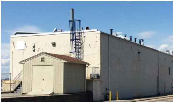
Photo: Existing Laboratory Building
