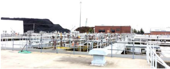
Photo: FP Blower Building
