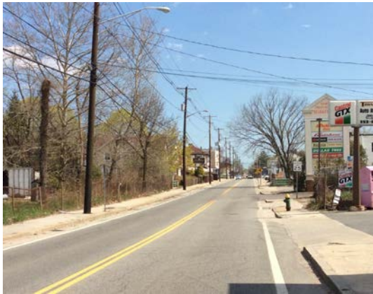
Photo: Branch Avenue Interceptor improvement location
