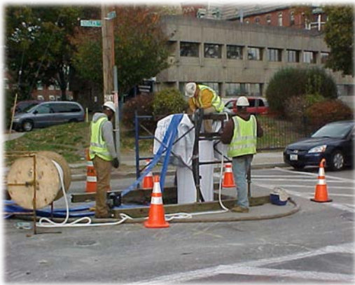
Photo: Lining at an interceptor improvement location
