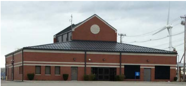
Photo: Tunnel Pump Station
