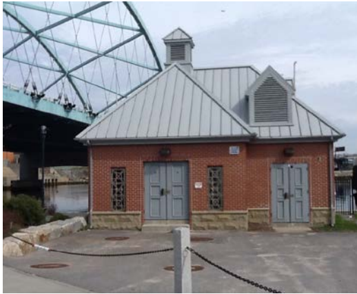
Photo: Providence River Siphon House
