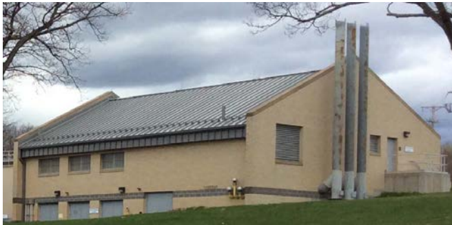
Photo: Bucklin Point Boiler Stacks
