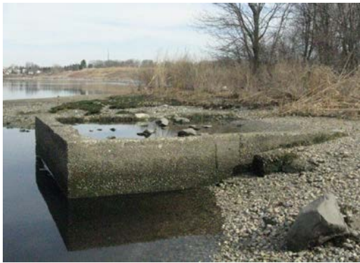
Photo: Bucklin Point WWTF Outfall
