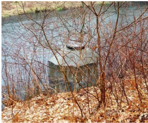
Photo: Manhole along river
