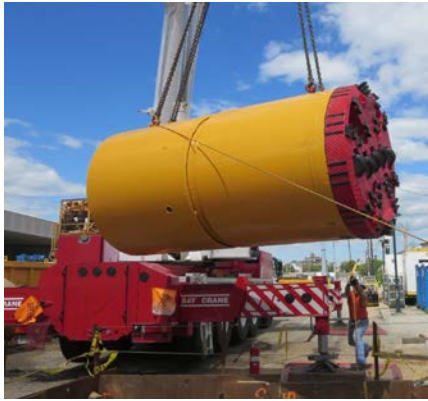
Photo: Micro Tunnel Boring Machine Installation
