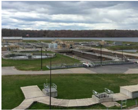
Photo: Bucklin Point WWTF
