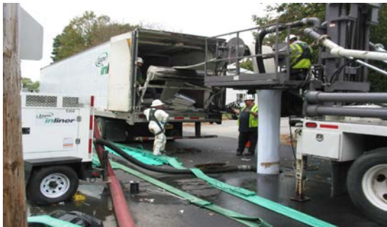
Photo: Conducting Sewer System Repairs
