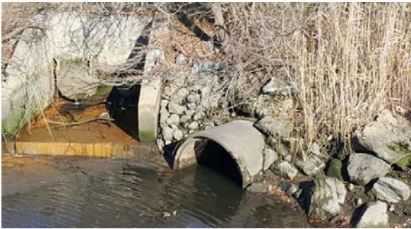
Photo: End of North Outfall Pipe
