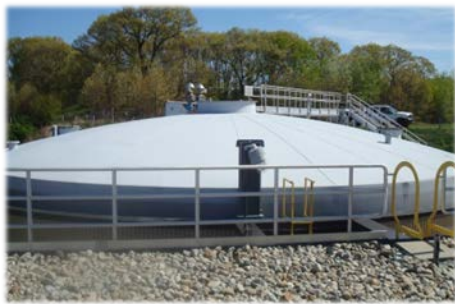
Photo: Bucklin Point Digester
