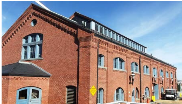
Photo: Existing Maintenance Building
