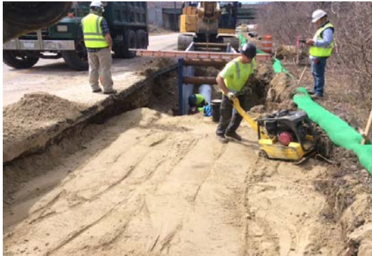
Photo: Construction on Greenville Avenue
