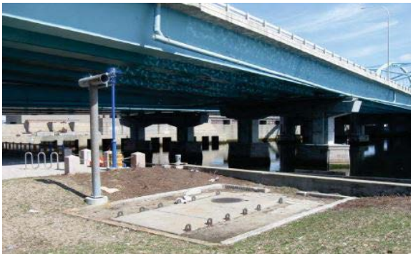
Photo: Siphon Outlet Chamber
