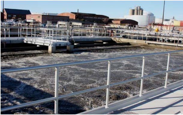
Photo: Aeration Tanks FPWWTF
