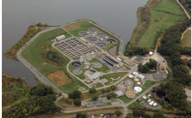
Aerial photograph of the Bucklin Point Wastewater Treatment Facility.
