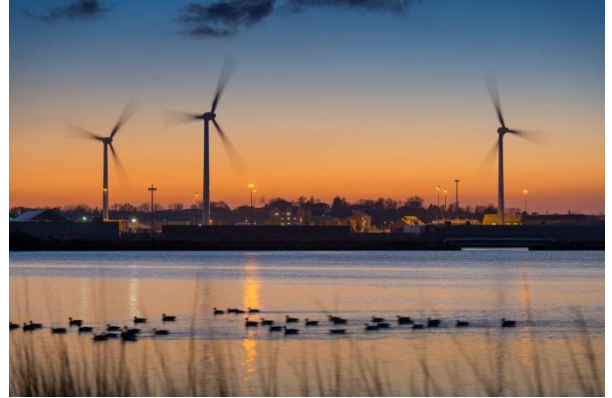
The three wind turbines constructed at Field's Point provide a grand statement and show NBC's strong commitment to the strategic goal of obtaining 100% of NBC's electricity needs from renewable sources.
