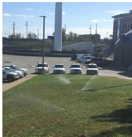
Irrigation systems operating at the Field's Point treatment facility utilizing recycled wastewater.
