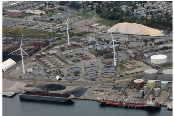
Aerial photograph of the Field's Point Wastewater Treatment Facility.
