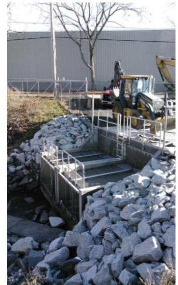
IM staff removing solid debris collected from a netting facility at the discharge of outfall #220 in Pawtucket.
