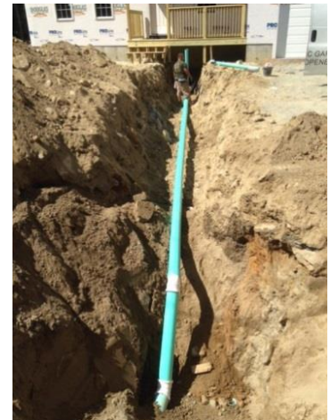
A residential sewer connection being installed in the NBC service district.
