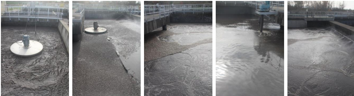
BNR facilities (pictured here at Bucklin Point) were installed at both facilities to meet new RIPDES permit requirements.
