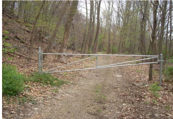
Photo: Newly installed barway gate for access to the BVI Easements
