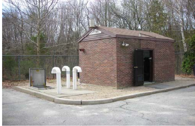
Photo: The Central Avenue Pump Station
