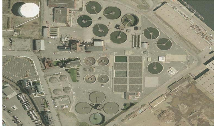
Photo: Aerial view of the FPWWTF
