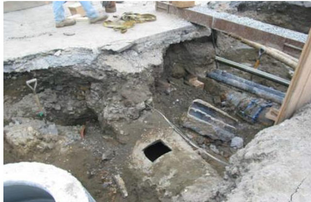
Photo: Removal of abandoned pipe at Atwells Ave. and Valley Street
