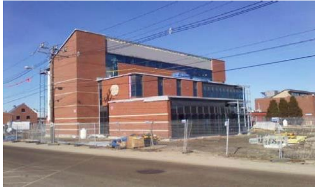
Photo: Newly constructed Operations building.
