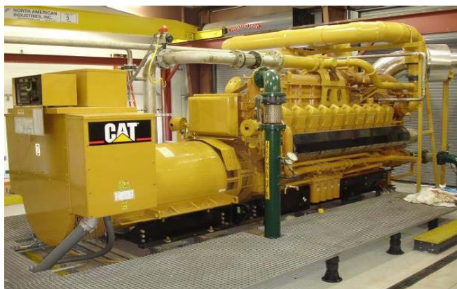
Photo: A Caterpillar reciprocating engine
