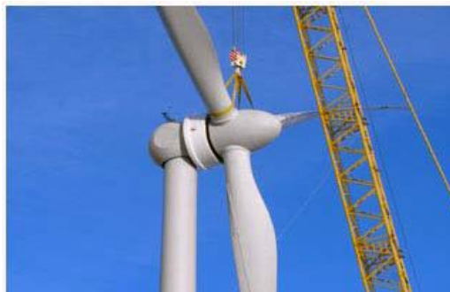
Photo: Assembly of a pre-built wind turbine
