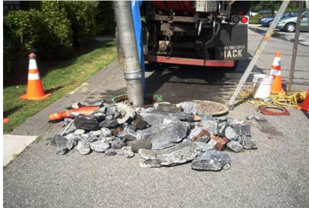
Photo: Heavy rock debris removed from sewer off Manton Ave
