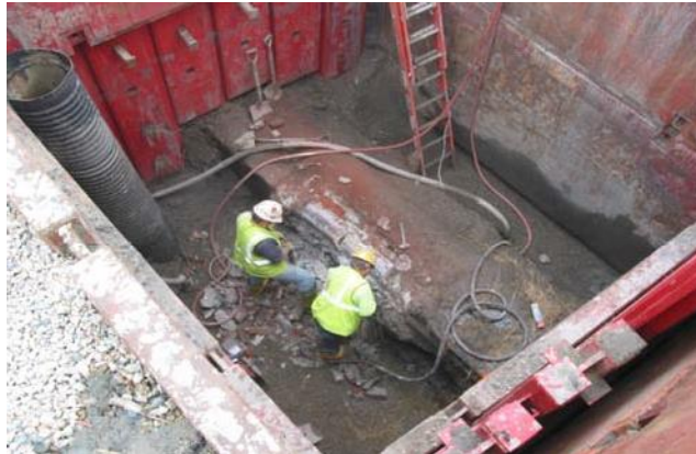
Photo: Removal of brick encased around an 8 inch pipe
